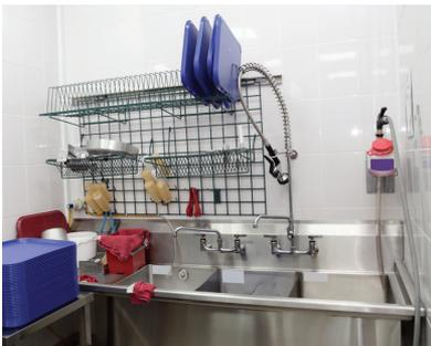
Dish cleaning offers opportunities for saving water as well. Before plates and dishes are loaded into the dishwasher they are often cleaned with a pre-rinse spray valve. Replacing an old pre-rinse spray valve, (which may use 2 to 5 gallons per minute) with an EPA WaterSense® labeled model using 1.28 gallons of water per minute will yield significant savings at a low cost.
