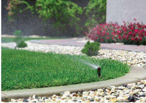
efficiency. If there is an automatic irrigation system in place it should be equipped with water savings devices and of course checked for leaks. Rain sensors, soil moisture sensors, and weather based irrigation controllers utilizing evapotranspiration information can be installed to prevent the irrigation system from operating when it is not needed. There may also be opportunities for rainwater capture and other types of on-site water reuse that can be used for irrigation.
