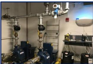
The New School implemented a reuse system at its Manhattan Campus University Center that collects rainwater, as well as water from sinks, showers, and washing machines to distribute for reuse in toilets, green roof irrigation, and the buildings cooling tower. This system helps cut potable water usage by 74% and reduces sewer discharges.
