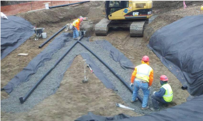
Construction of the tiered bioretention facility at Shoelace Park, completed in 2012. Monitoring activities during 2013 will evaluate pilot performance.
