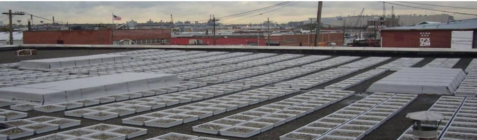
On a roof along Metropolitan Avenue, a system of trays manages over 300,000 gallons annually.
