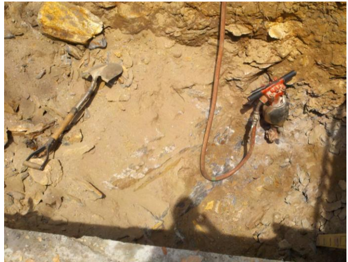
Subsurface conditions below the south parking lot system consist mostly of clay and large rocks.
