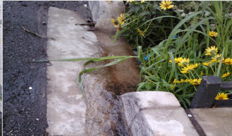
Vegetation at an enhanced tree pit at Blake Avenue (left), which has modified open curb cuts (right) to capture stormwater runoff.
