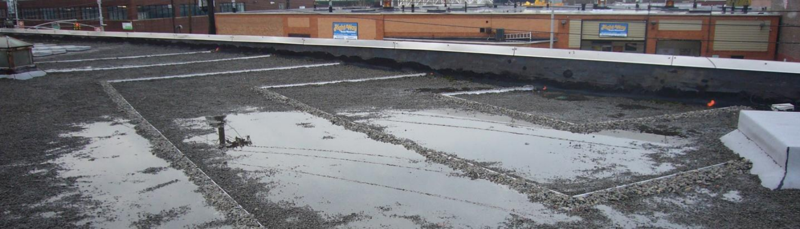
At the Metropolitan Avenue pilot, three variations on blue roof designs are being monitored: modified inlet, check dams, and tray systems. Specially designed inserts were installed inside existing drain pipes in order to measure outflow.
