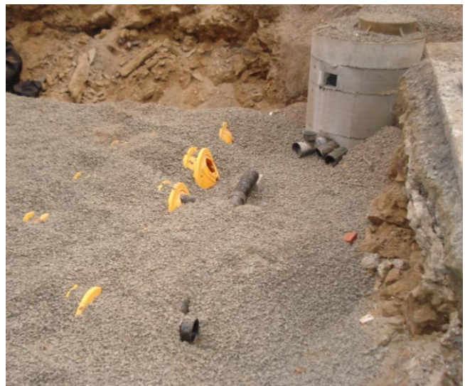
Construction of the north parking lot subsurface system.
