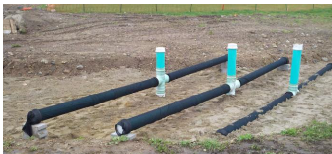
Infiltration wells at North and South Conduit Avenues bioretention prior to bioretention soil installation. These wells capture water that has infiltrated through a depth of soil.
