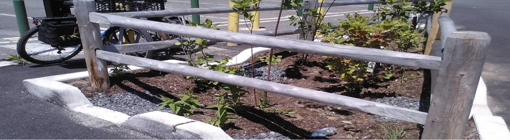
One of three constructed bioretention facilities with curb inlets in the Canarsie Parking Lot.
