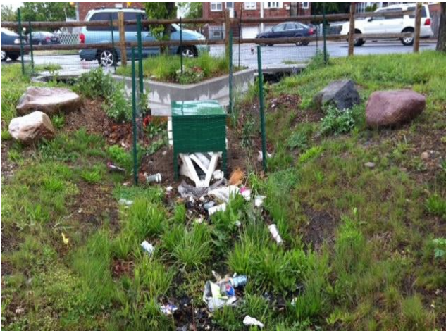
An example of litter and debris flowing from the curb cut inlets.
