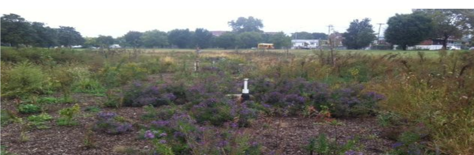
Vegetative growth and root development at the bioretention facility at North and South Conduit Avenues may be contributing to increased infiltration rates between 2011 and 2012.
