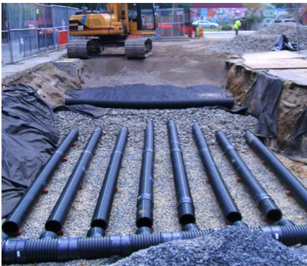
Construction of the south parking lot subsurface system.
