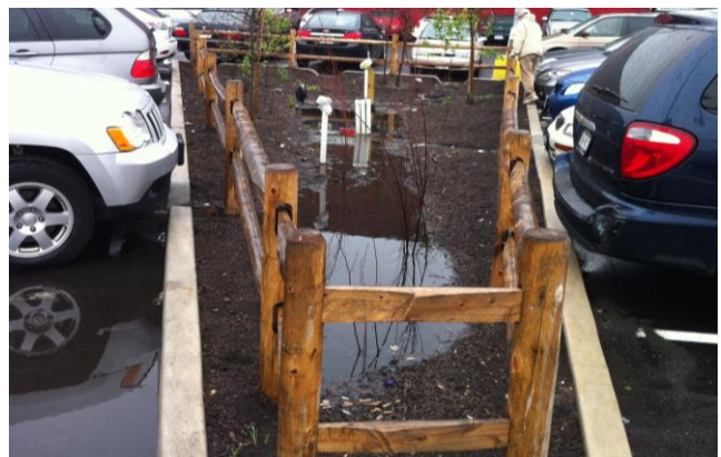
Ponding in one of the bioretention areas following a storm event.
