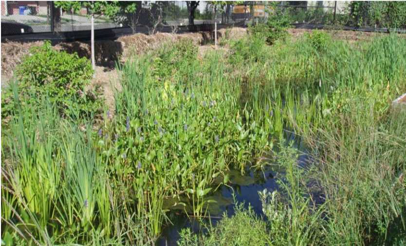
Established vegetation in the wet meadow pilot at the Spring Creek MTA Bus Terminal under saturated conditions. Monitoring equipment was installed at the outlet (shown on right) to measure outflow.
