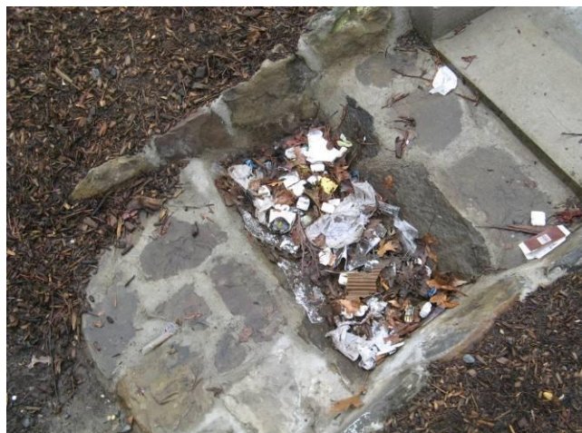
Litter and debris captured by a bioretention curb cut inlet sump, which consolidated maintenance activities.
