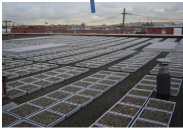
The rooftop was partitioned to examine three types of blue roofs and an uncontrolled reference area.
