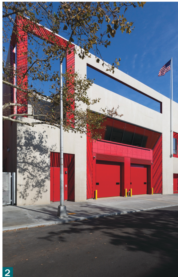
1. and 2. Construction of a firehouse, Rescue Company 2, Sterling Place between Howard Avenue and Saratoga Avenue, Brooklyn; Department of Design & Construction
