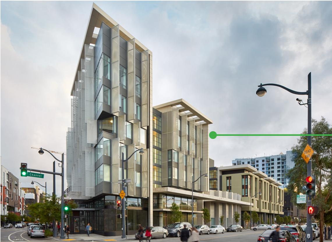
vertical solar shades provide visual interest and protect against interior heat gain
