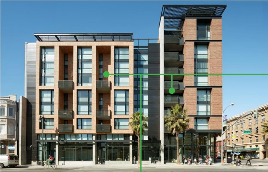
varied balcony design that is integrated into the overall massing and provides per-floor and per-unit access
