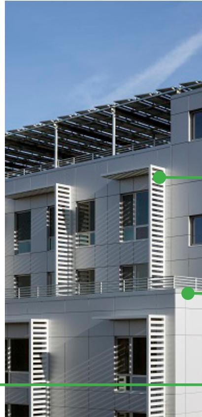
solar screens to mitigate heat gain within units
