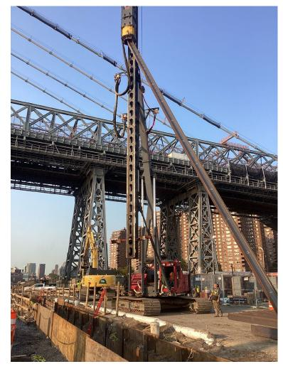
H-pile installation for deep sewer work – September 2022
