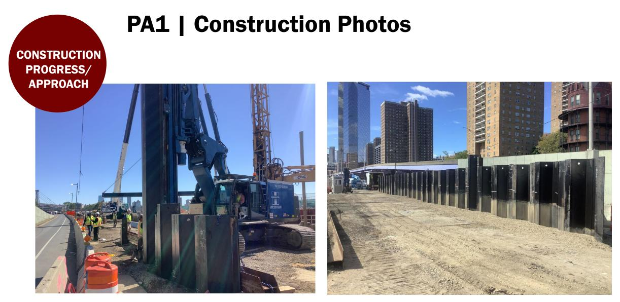
Sheet Pile installation for floodwall along the Greenway with vibrating pile rig – September 2022
