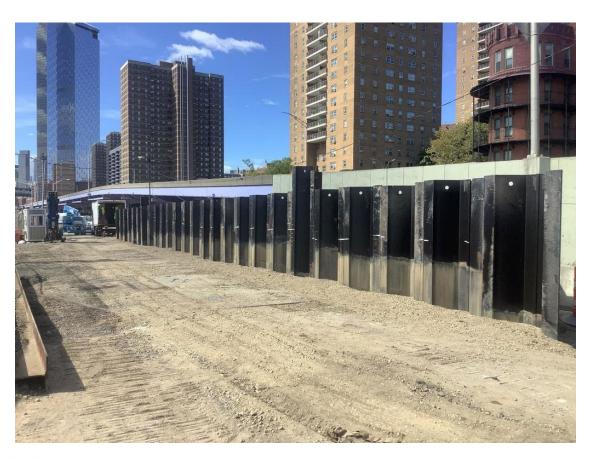
Sheet Pile installation for floodwall along the Greenway with vibrating pile rig – September 2022
