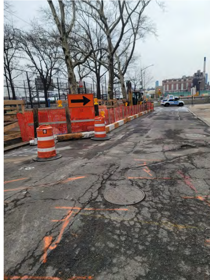
Storage area on Jackson St. - February 2023
