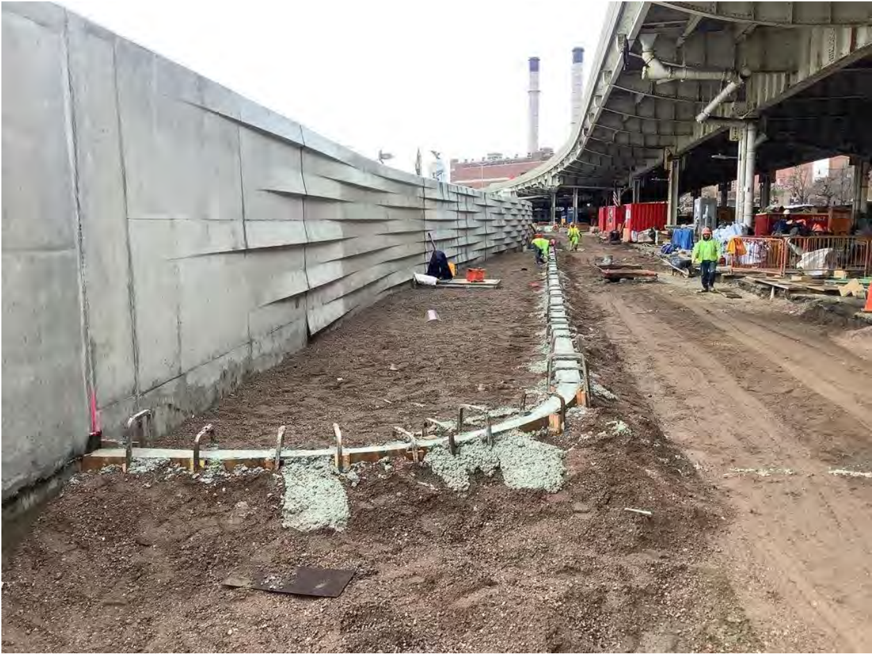
Greenway curb install south of E20th Street - February 2023
