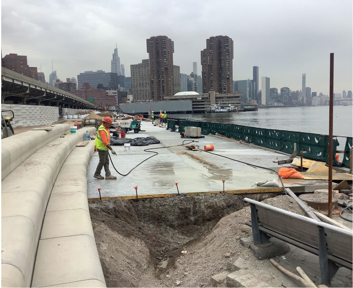
Stuyvesant Cove Park south restoration - February 2023
