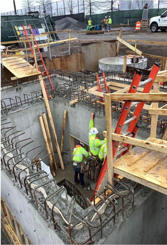
Sewer Chamber - February 2023
