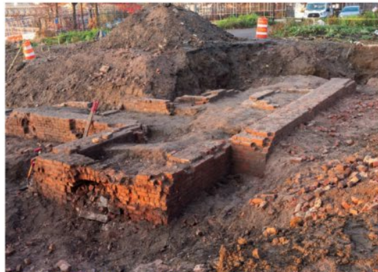
View to southwest showing re-used and partially abandoned iron foundry remains, with chimney base in foreground.
