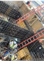
PA1 Construction, January 2023
