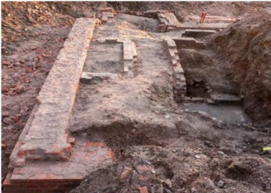
View to east of sugar refinery/iron foundry walls. The north foundation of the factory is at left. The rectangular area at top is an apparent chimney base. A bluestone walkway is exposed at right.
