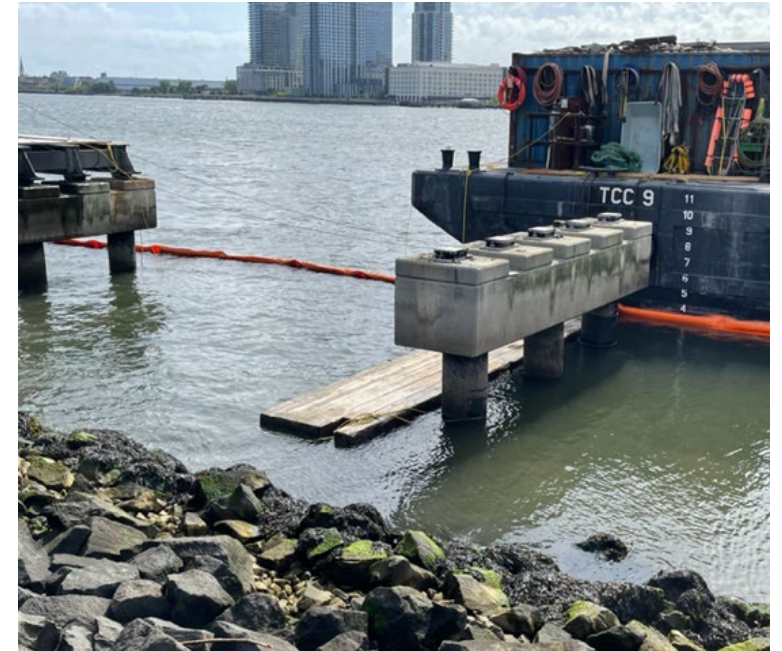
Turbidity Curtain at removal of Embayment Esplanade
