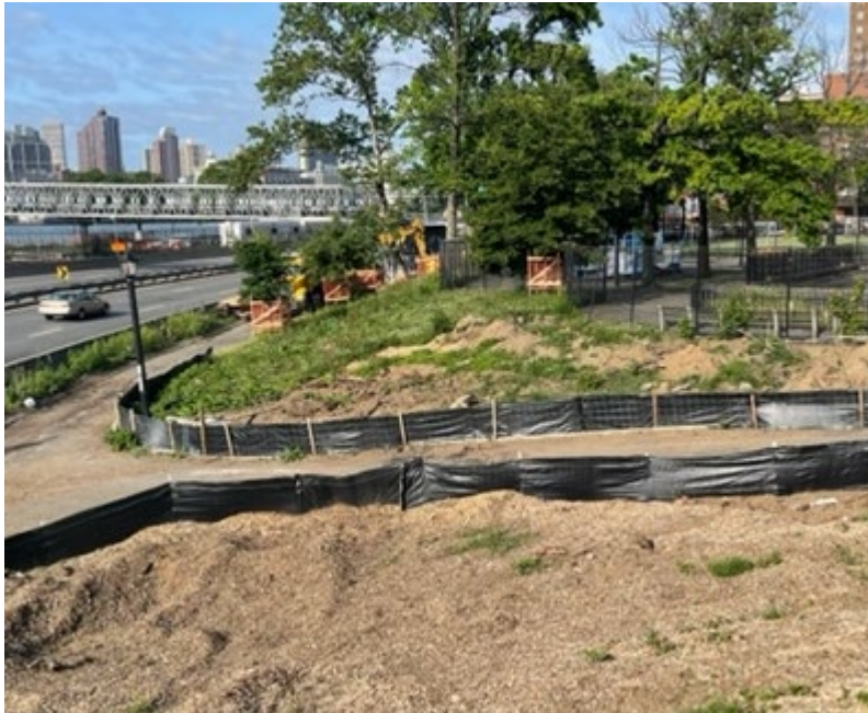
Silt Fence at Corlears Hook Park
