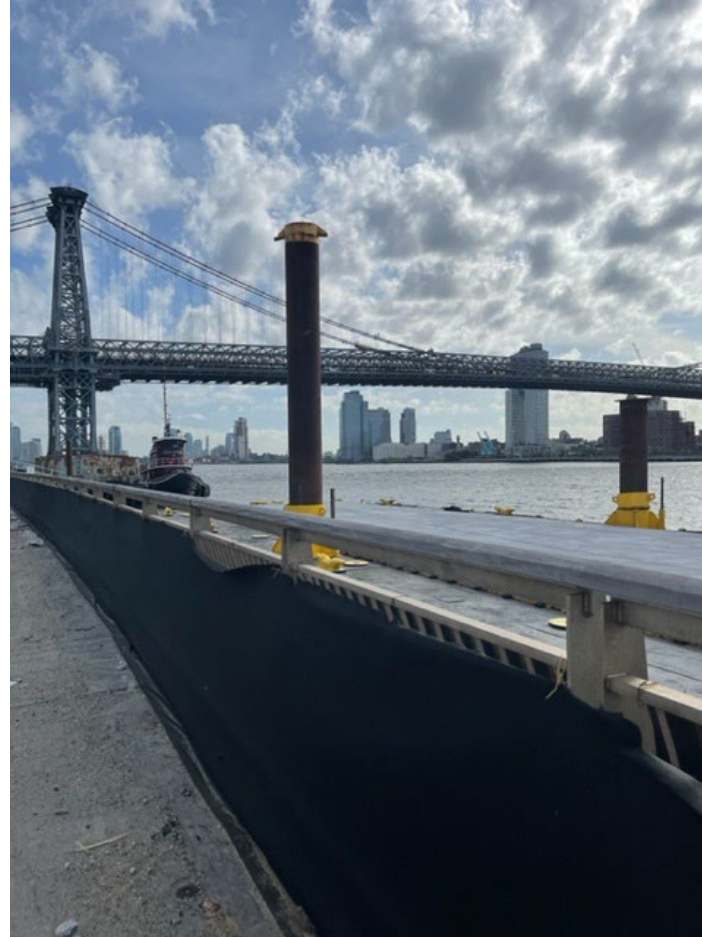
Silt Barrier along Esplanade
