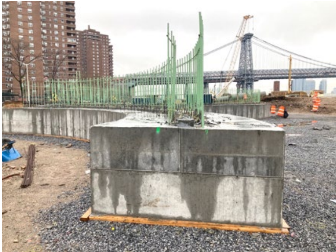
Corlears Hook Bridge East Abutment - January 2023
