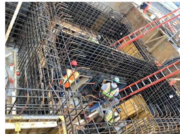
Deep Sewer Excavation and Construction - January 2023
