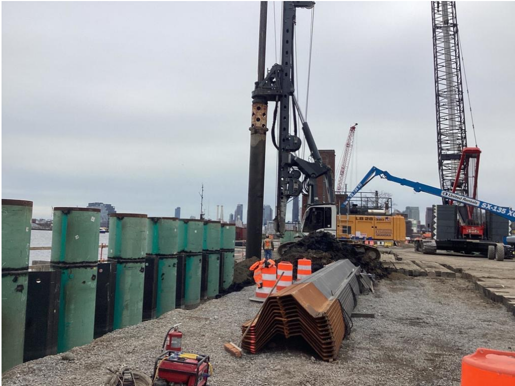
Combi-wall construction – April 2023
