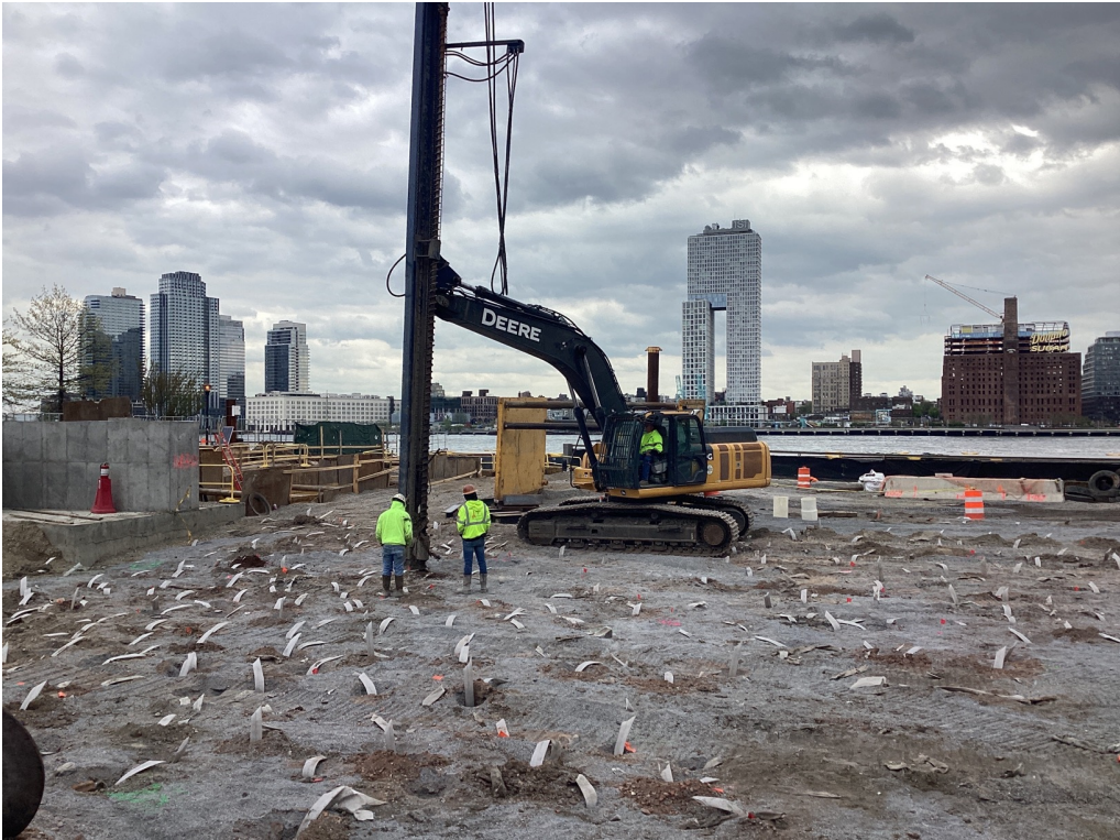
Wick drain installation – April 2023
