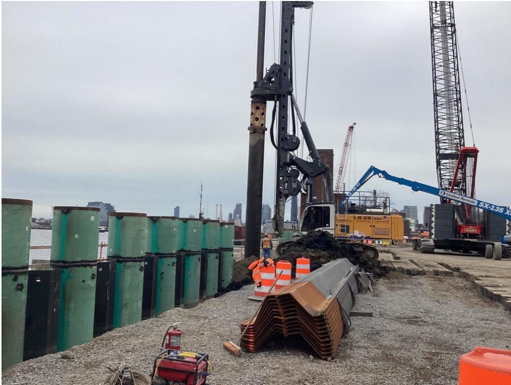
Combi-wall construction – April 2023
