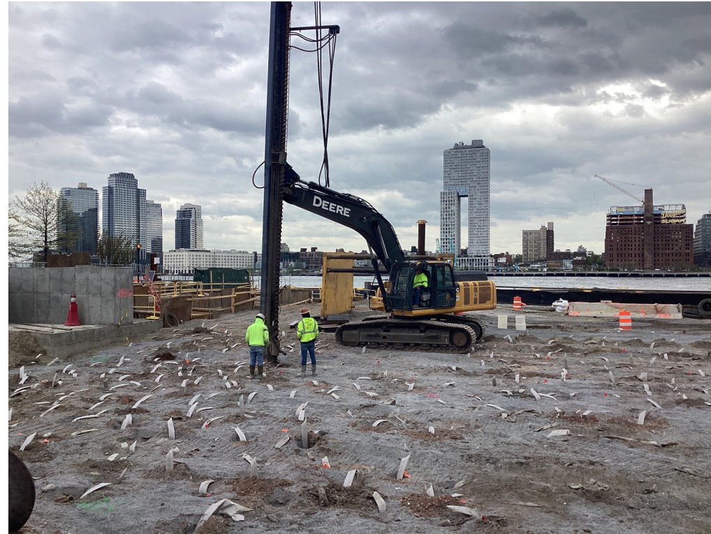
Wick drain installation – April 2023
