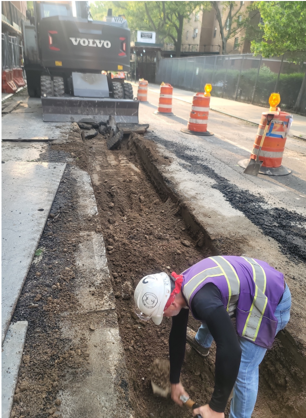
Excavation for Water Main - May 2023
