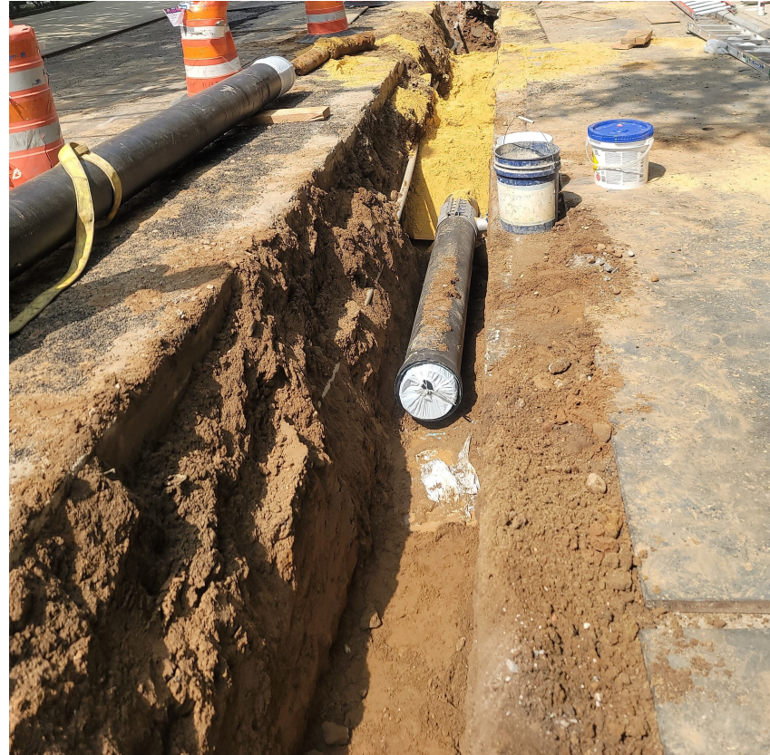
New 12" Distribution Water Main - May 2023
