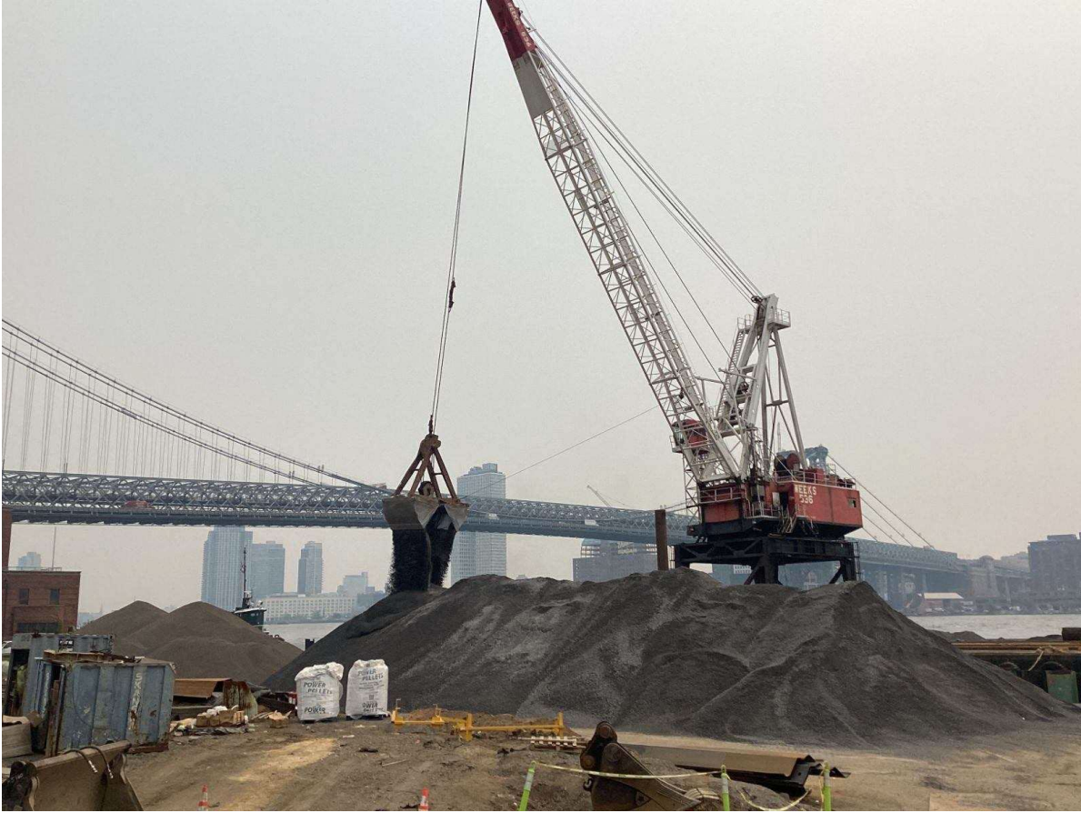
Delivery of fill material by barge – June 2023
