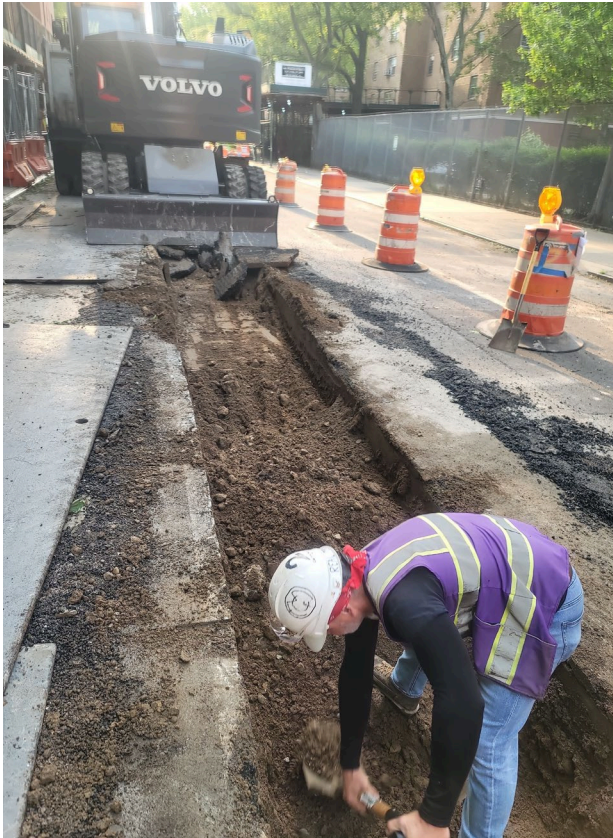
Excavation for Water Main - May 2023
