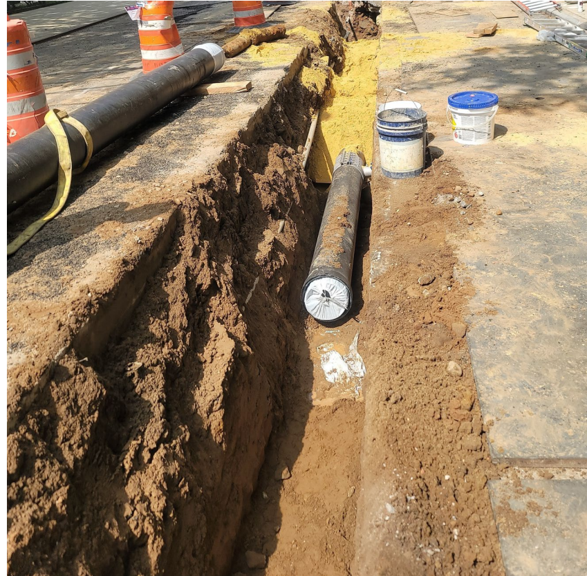
New 12" Distribution Water Main - May 2023
