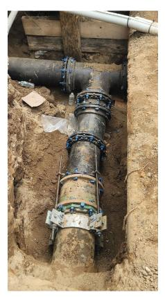
Installation of 12" Water Main, Intersection of Water St. and Jackson St. - July 2023
