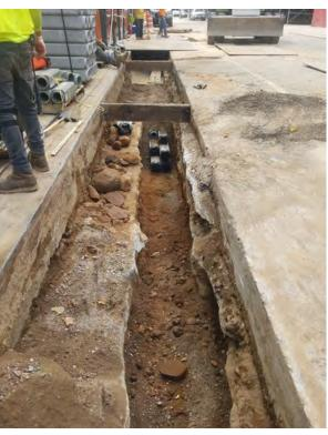
ConEd conduit installation on Water St. - August 2023
