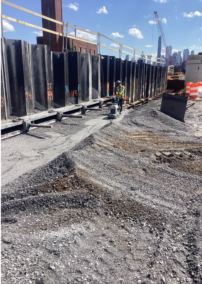
Backfilling Operations - August 2023
