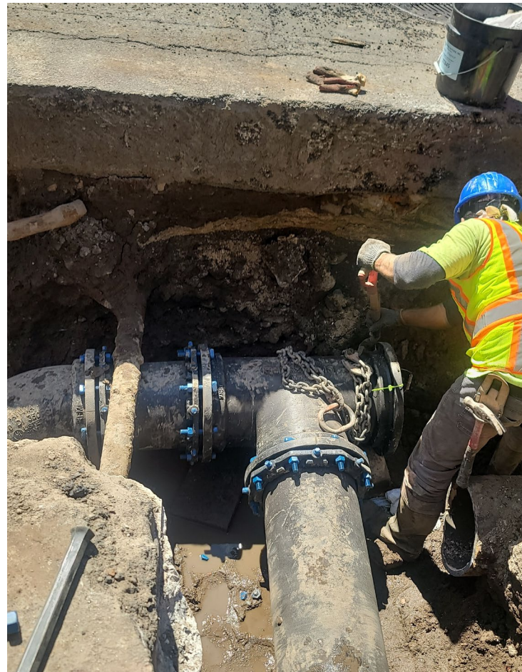
12"x12" Three-way installation on South St & Gouverneur Slip – September 2023
