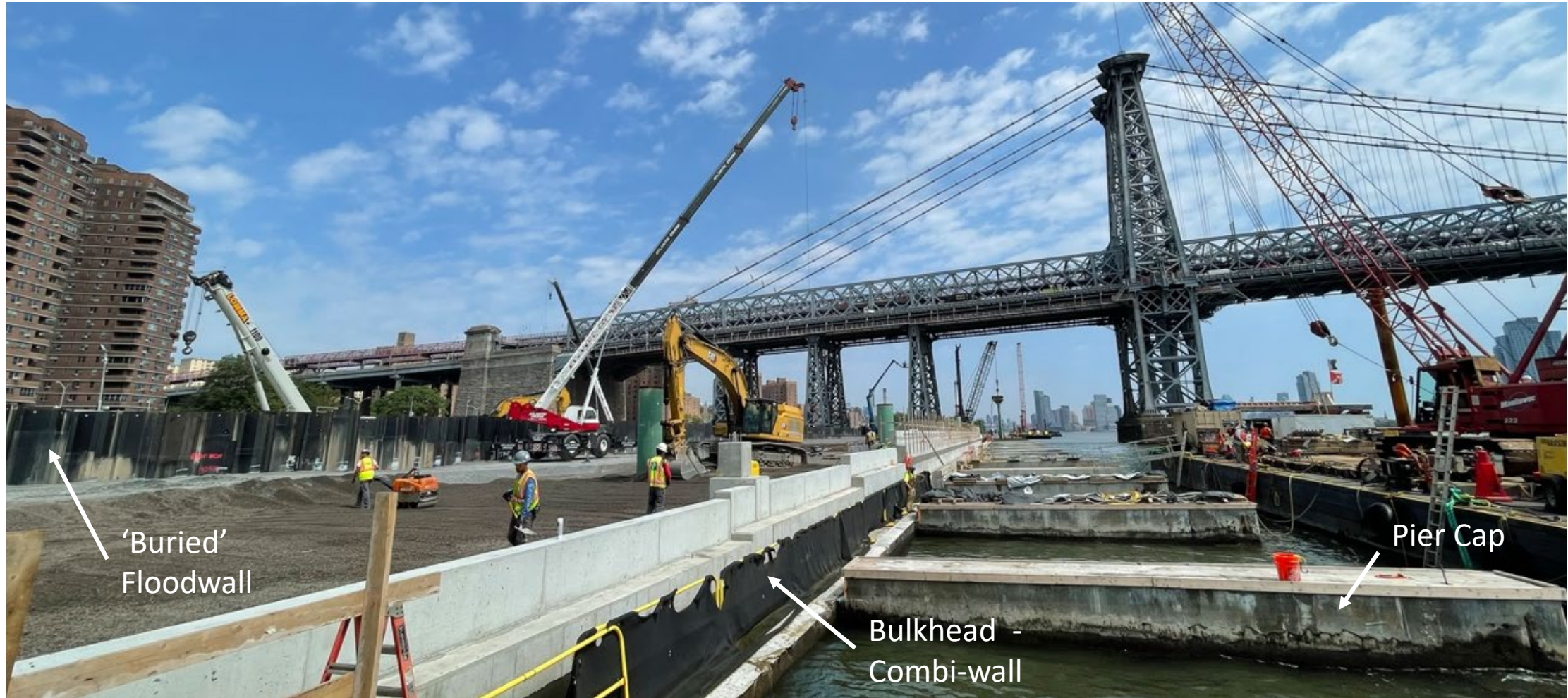
Future Buried Floodwall near Williamsburg Bridge - July 2023
