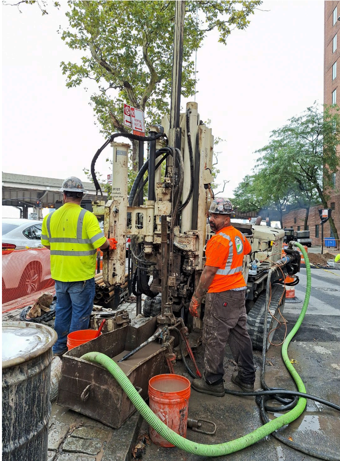
Field Investigation to locate existing interceptor sewer on E 20 St. – September 2023
