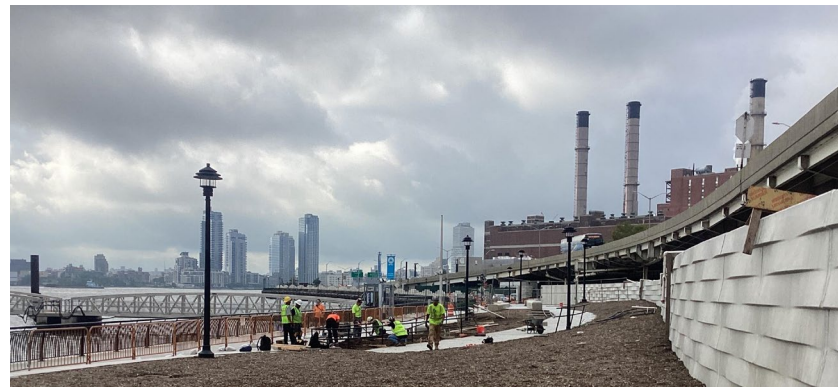
Stuyvesant Cove South Topsoil & Sea Rail Installation - August 2023
