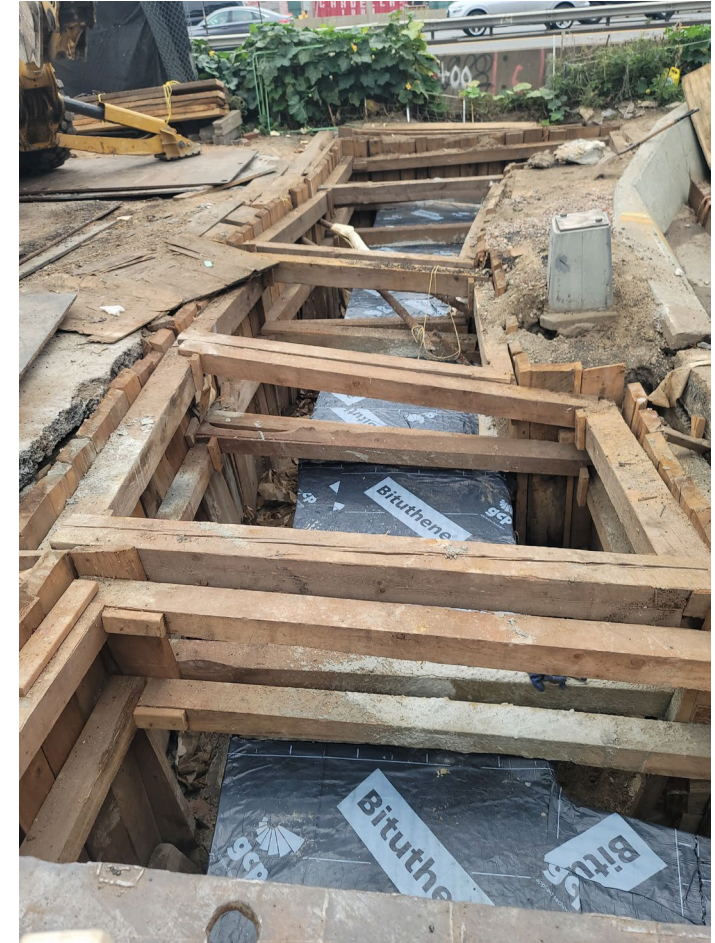
24" Steam Main New Casing & Water Proofing on Jackson St. – September 2023
