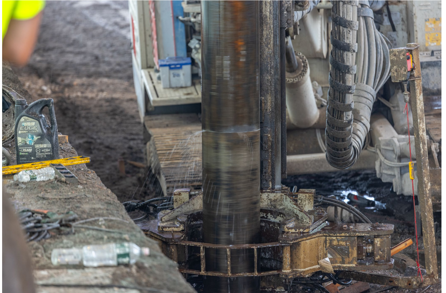
Micropile Installation – September 2023
