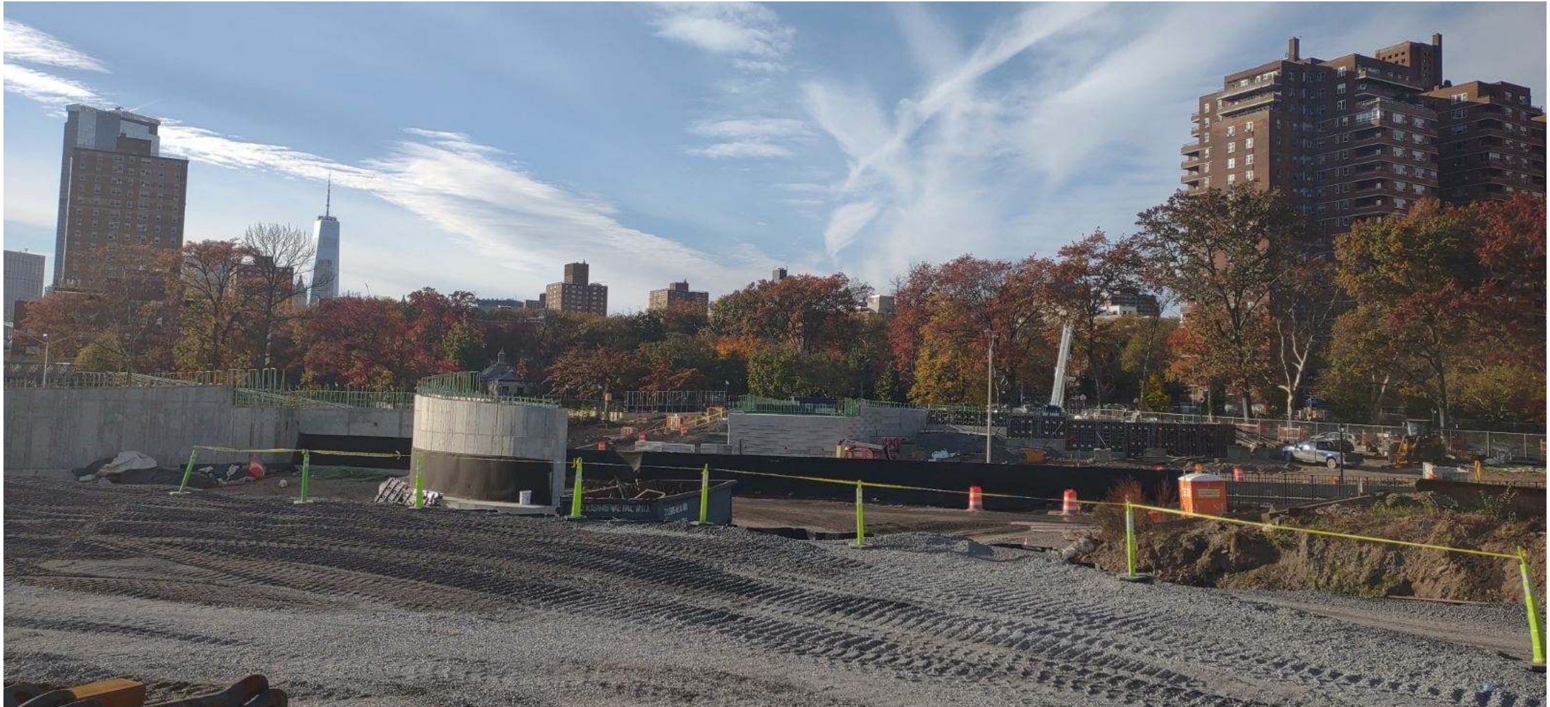
Corlears Hook Bridge Abutment Construction - November 2023
