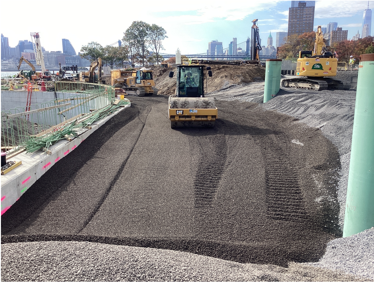
Lightweight backfilling by combi-wall at Embayment - November 2023
