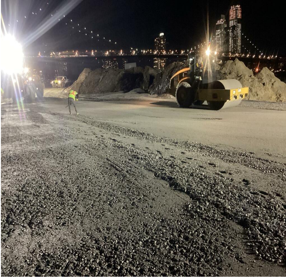
Lightweight backfilling Night Operations - November 2023
