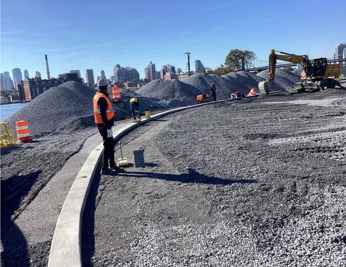
Ballfields 1 and 2 Construction - November 2023
