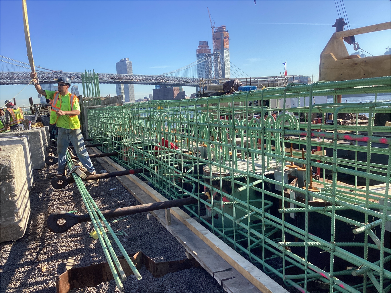
Combi Wall with rebar - October 2023
