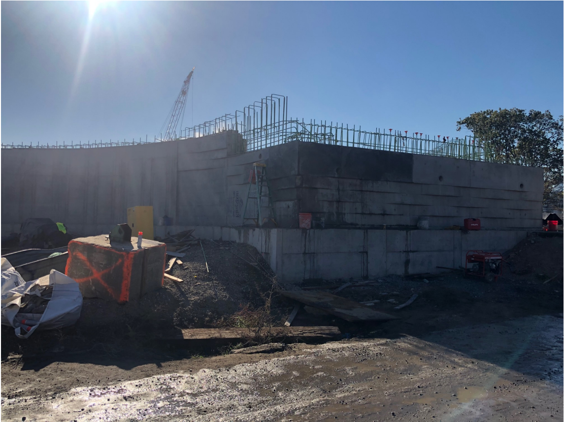
Eastern Corlears Hook Bridge Abutment - October 2023
