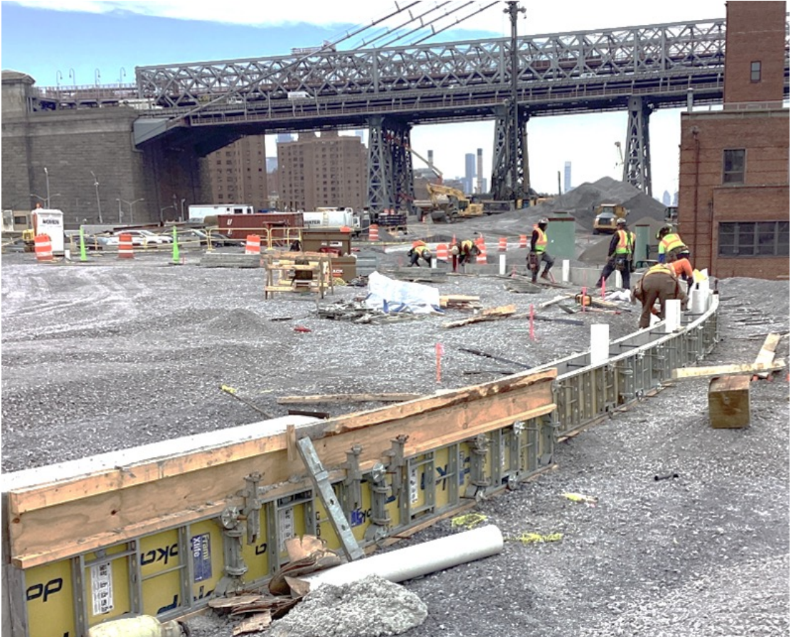
Ballfields 1 and 2 Curb Construction - October 2023
