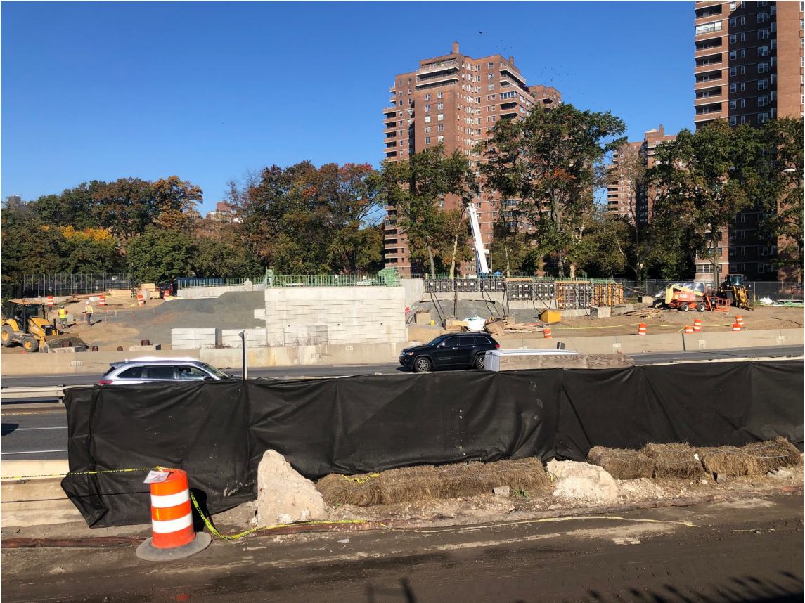
Western Corlears Hook Bridge Abutment Construction - October 2023
