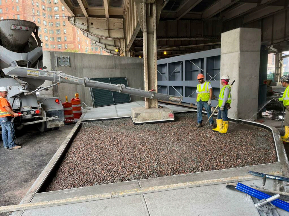
Sidewalk Restoration at Gate 10 - August 2023
