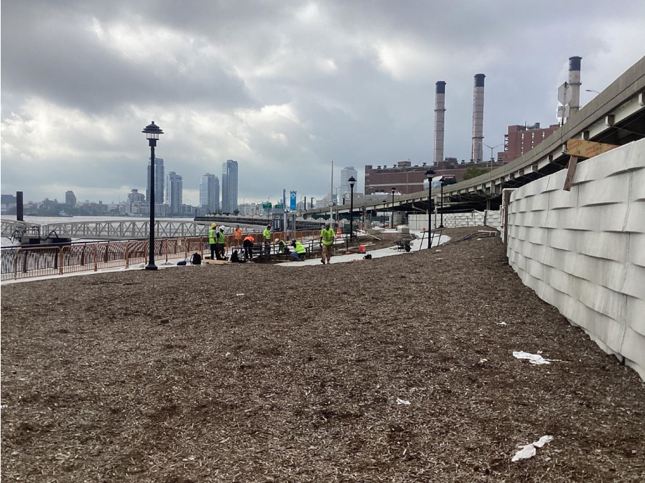
Stuyvesant Cove South Topsoil & Sea Rail Installation - August 2023
