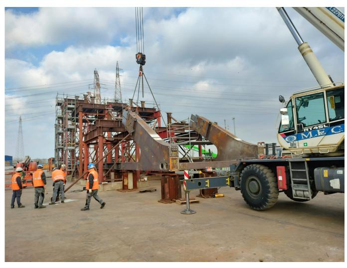
Test fit of Delancey Street Bridge superstructure at fabrication facility - November 2023
