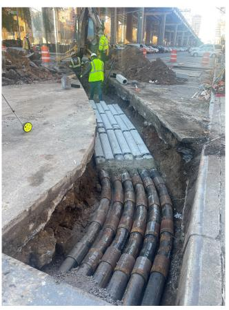
ConEd ducts installation in Delancey St. North by Lewis St. – November 2023
