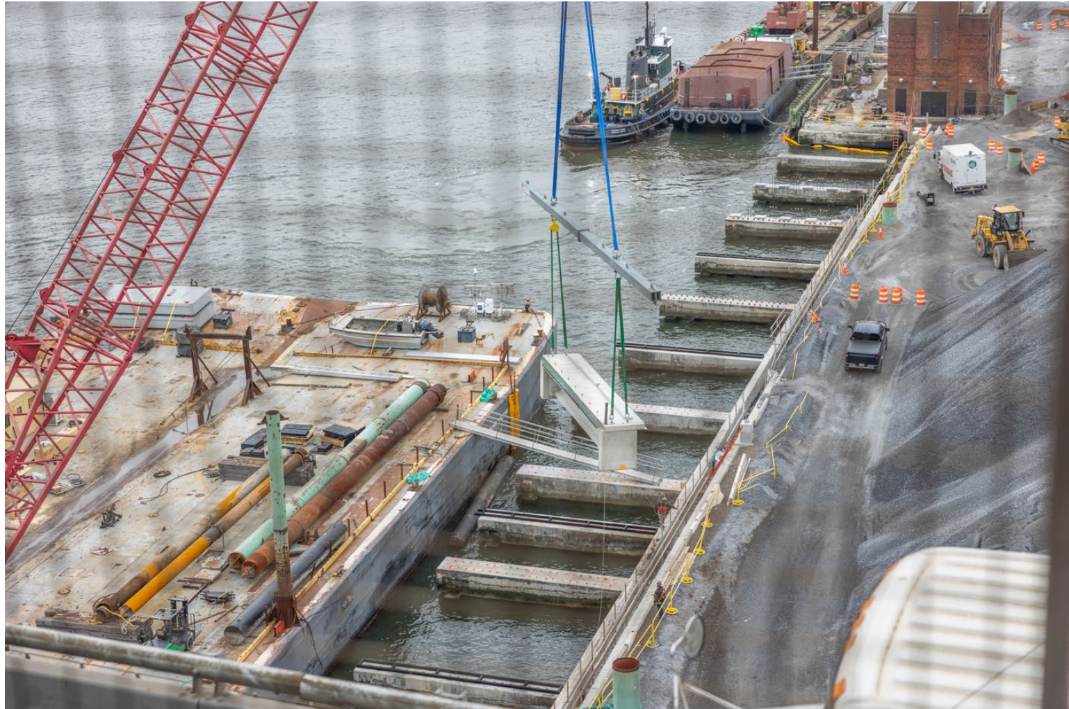
Placement of precast esplanade pieces by crane from barge - December 2023
