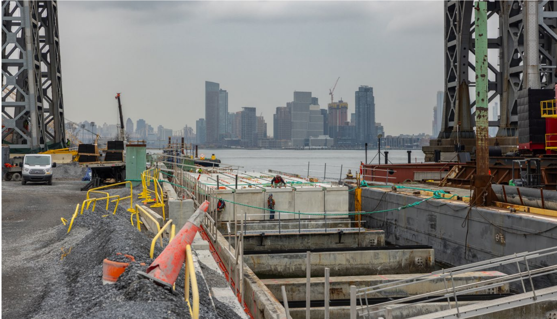
Placement of precast esplanade pieces - December 2023
