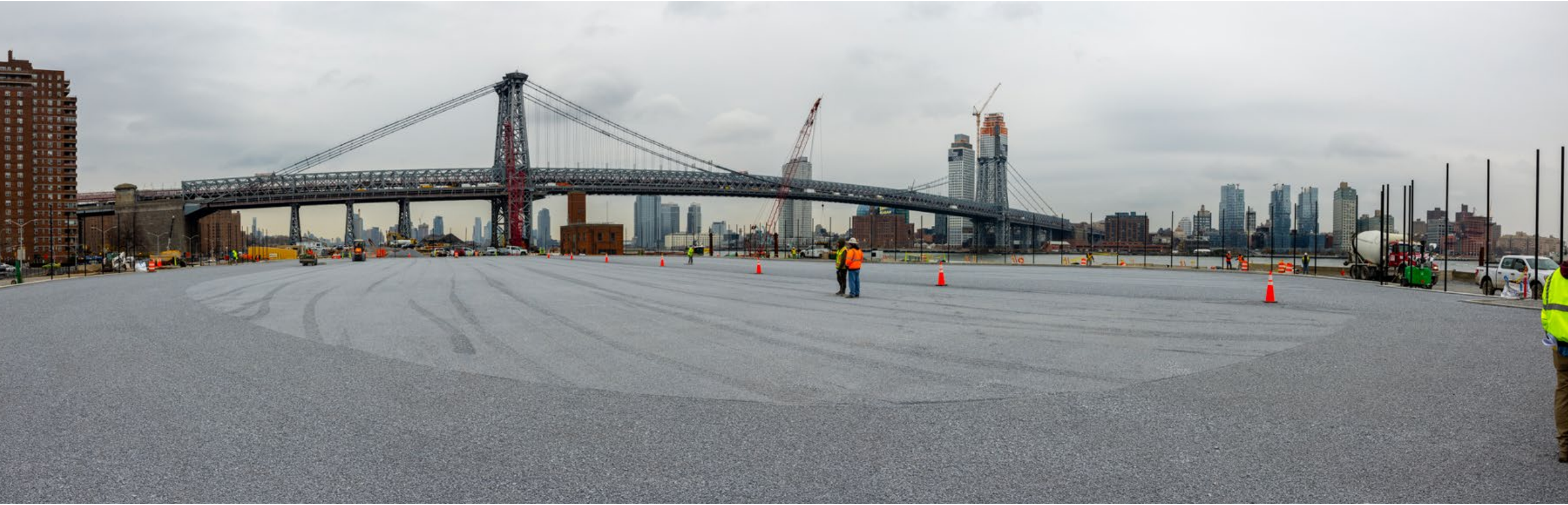
Ballfields 1 and 2 Construction - December 2023
