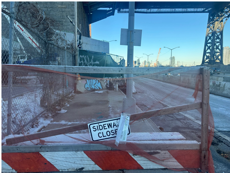
Before: Closed FDR Service Road Sidewalk – January 2024
