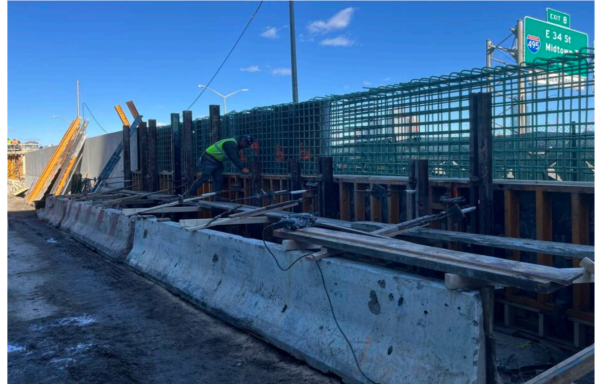
Floodwall reinforcement and form work near ConEd Generation Plant – February 2024
