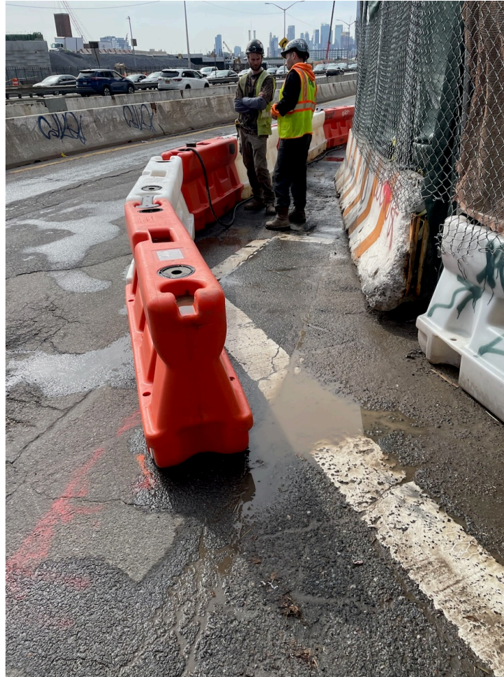
After: New pedestrian path at Delancey and FDR Service Rd – March 2024
