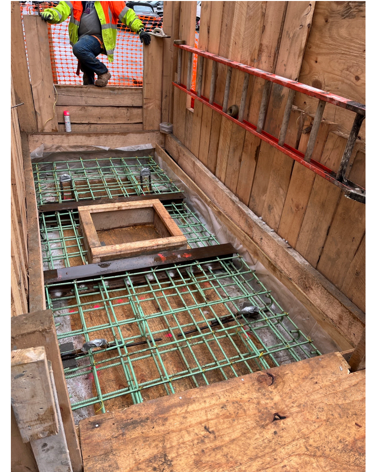
Manhole installation on Delancey St. N. - February 2024
