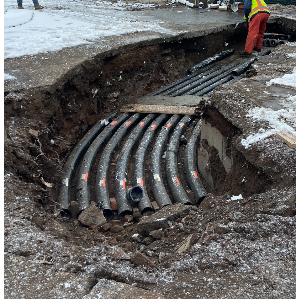
5" Conduit Installation in Jackson Street - February 2024
