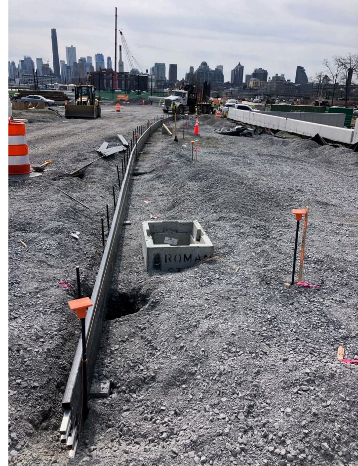
Future curb for Shared Use Path adjacent to M&O area – March 2024
