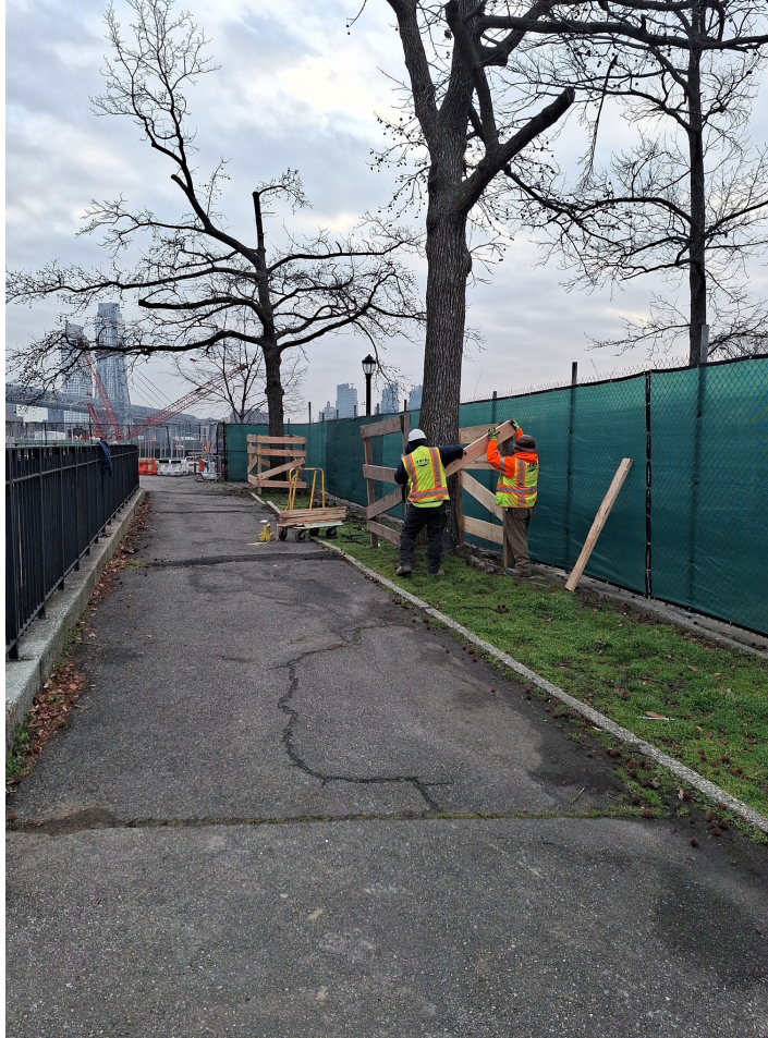
Staging and installation of tree guards - February 2024
