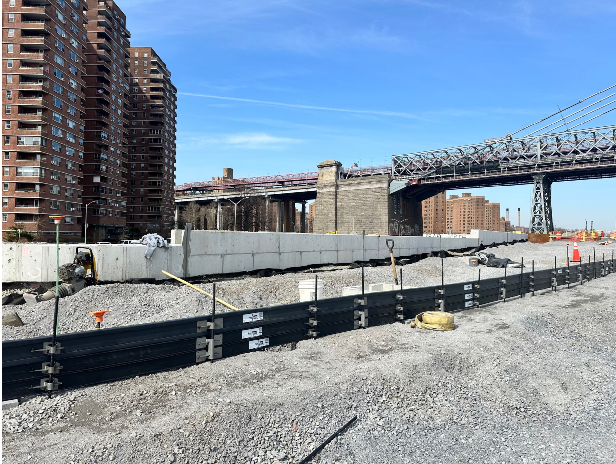
Future curb for Shared Use Path adjacent to M&O area – March 2024
