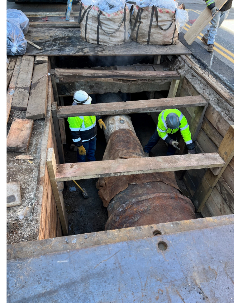
Steam main abatement E20th St. - March 2024
