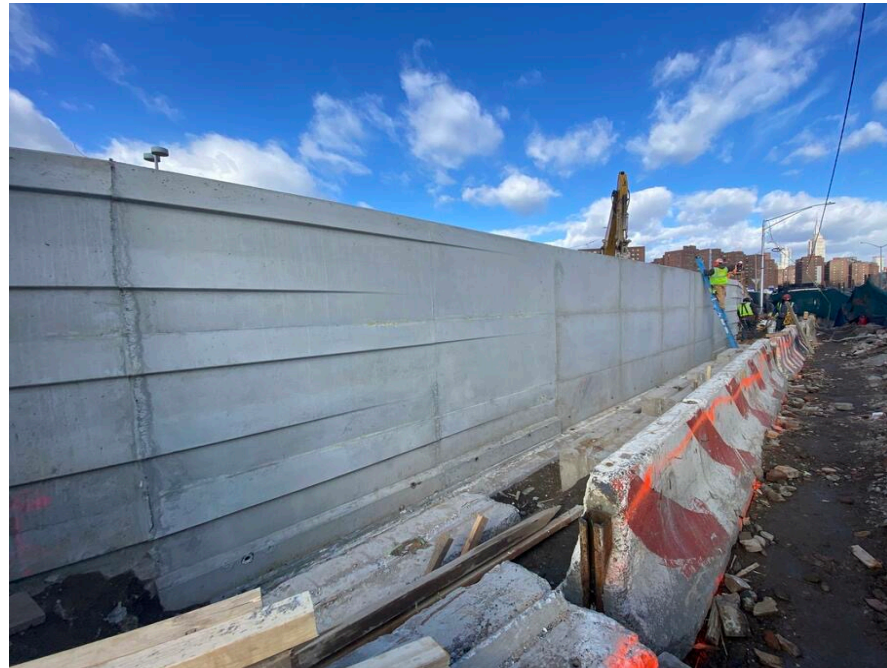
Bulkhead 1 Wall Monolith – March 2024
