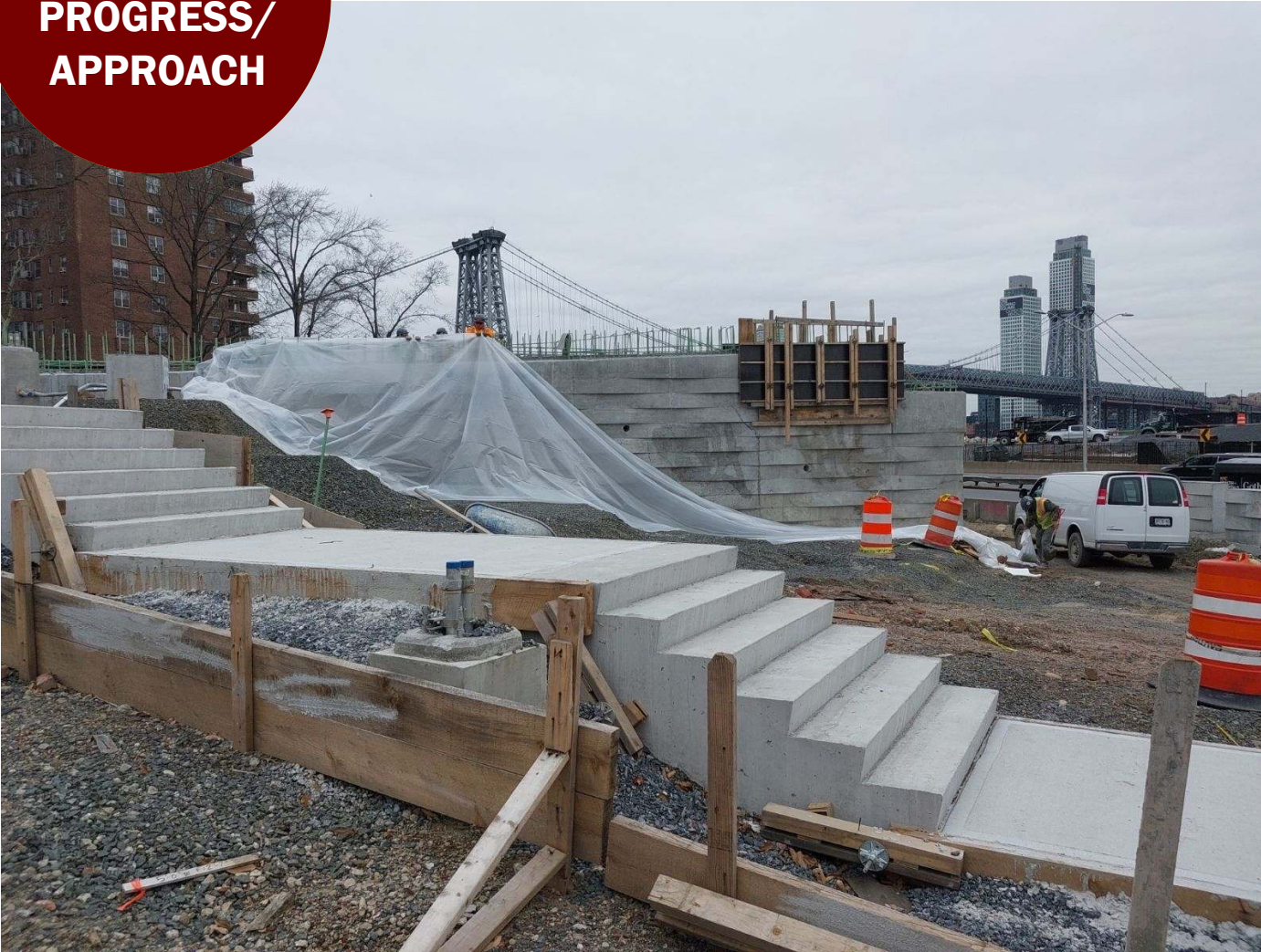
Stairs and retaining wall in Corlears Hook Park – March 2024
