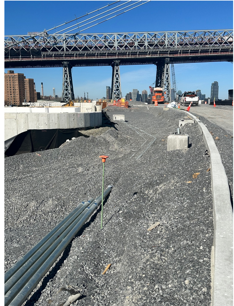
Shared use path curb near Parks M&O retaining wall. – March 2024
