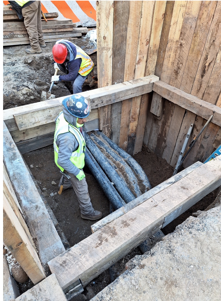
Sewer Test pit on Jackson Street - March 2024
