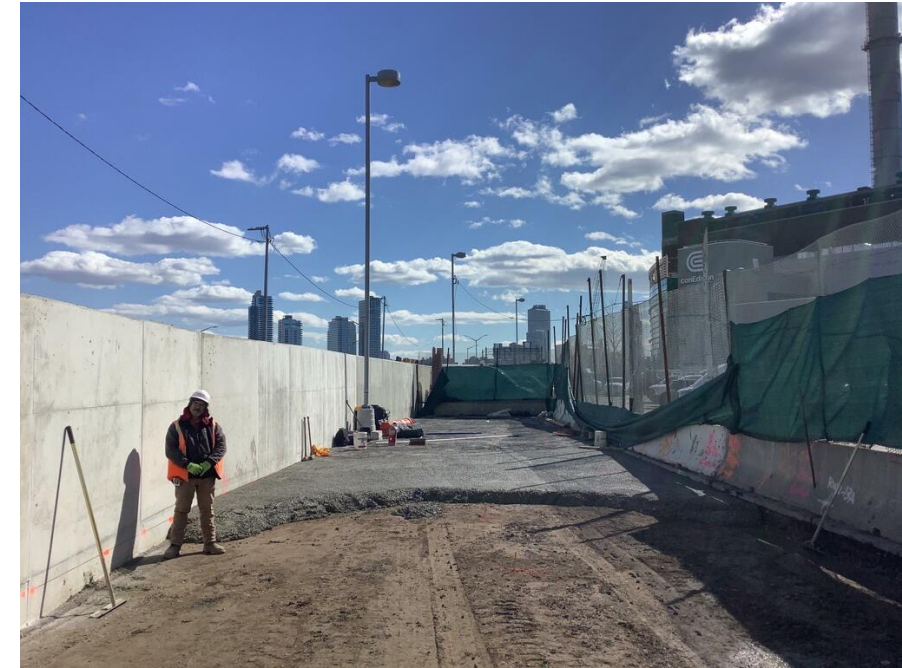
Restoration of Con Edison Parking Area – March 2024
