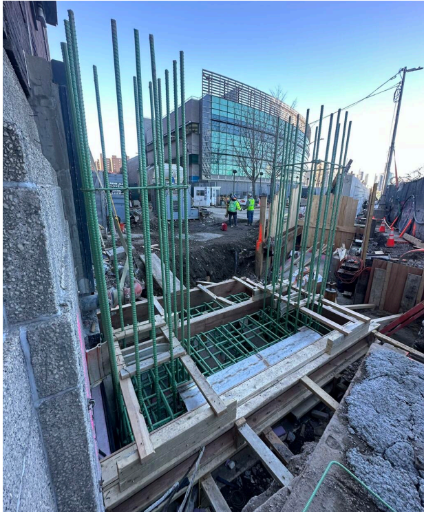
Gate 7 Foundation & Column Reinforcement – March 2024
