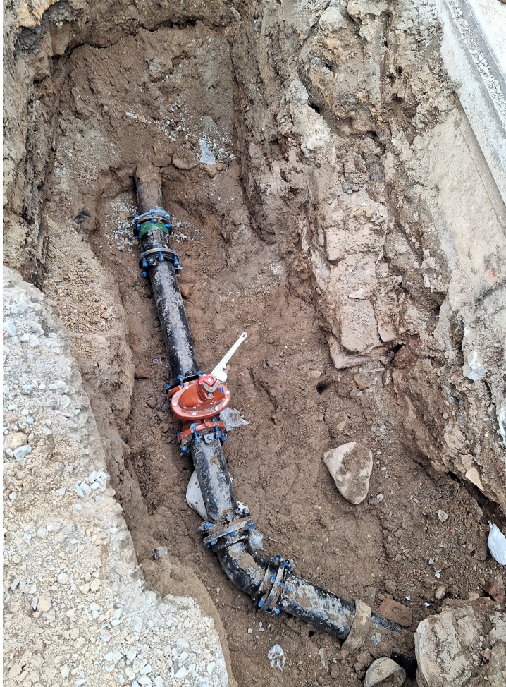
New Corlears Hook Park distribution water main connection - March 2024
