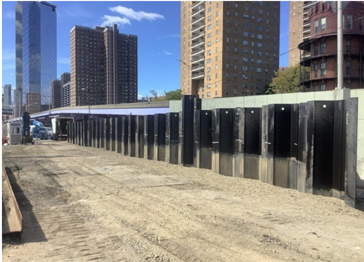
Sheet pile, Combi Wall, Sewer expansions
