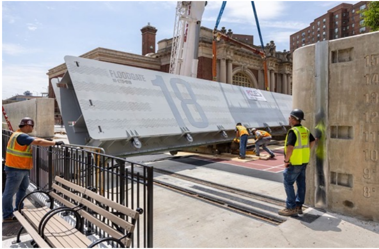
Floodgate, Asser Levy Playground, Flood wall
