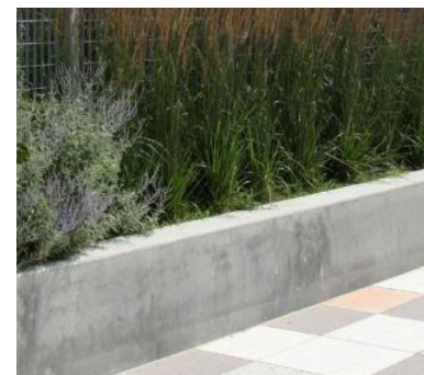
C.I.P. CONCRETE SITE WALLS
