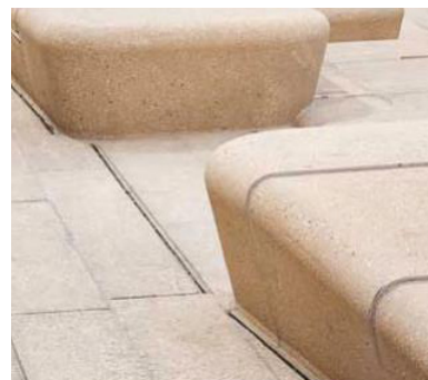
PRECAST CONCRETE SEATWALLS
