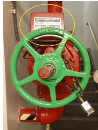
Tamper switch on a sprinkler valve
