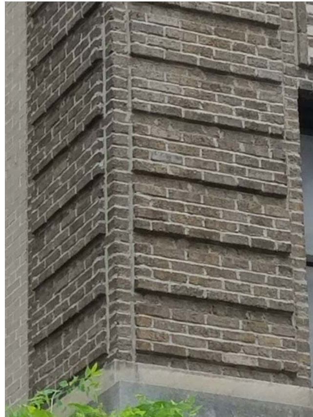
BRICK CORBEL CORNER
