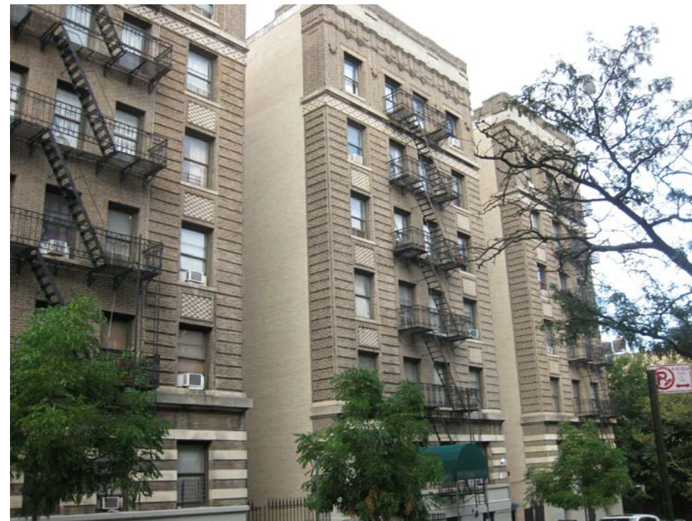
CONTEXT: BRICK CORBELING ON UPPER FLOORS ALTERNATING WITH STANDARD RUNNING BOND
