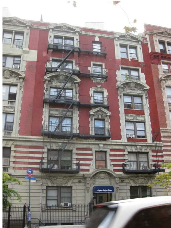
CONTEXT: WINDOW PANEL WITH BLACK WINDOWS AT 853 NICHOLAS AVE.
