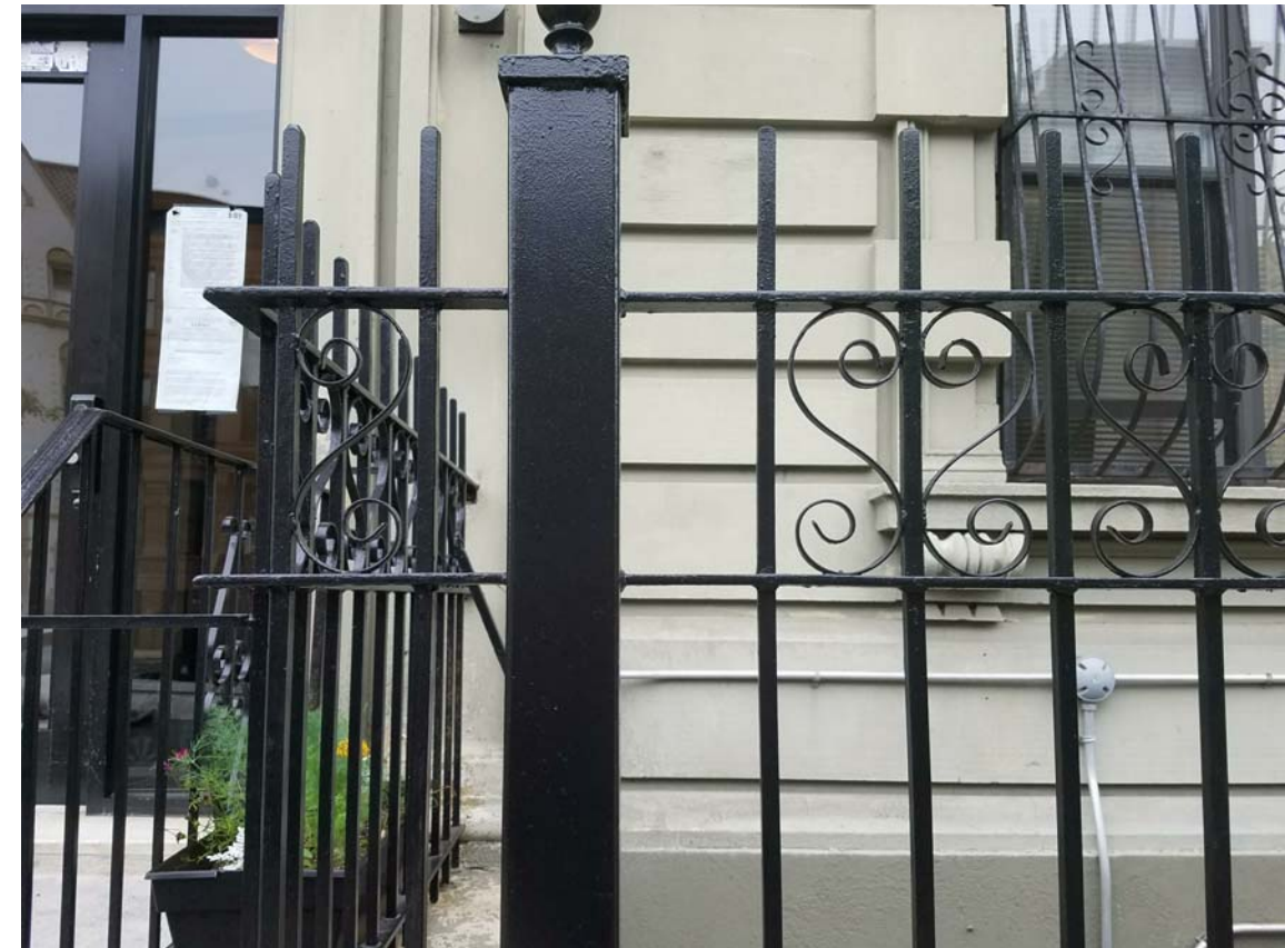
RAILING WITH DOUBLE HORIZONTAL BAND
