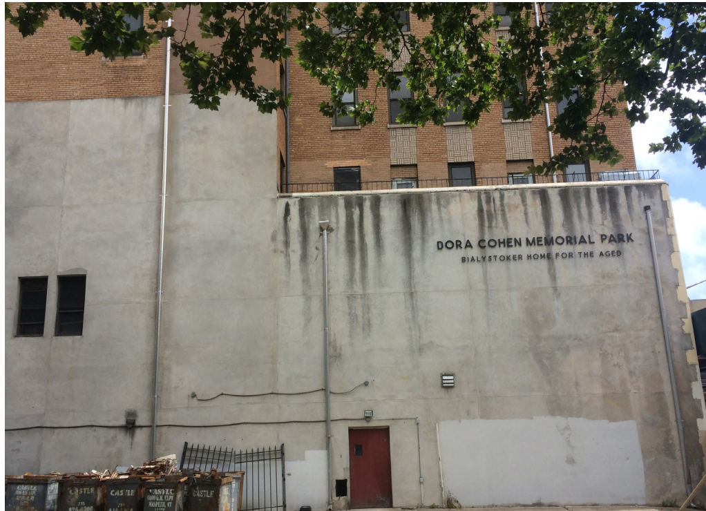
Exposed West Facade at Base
