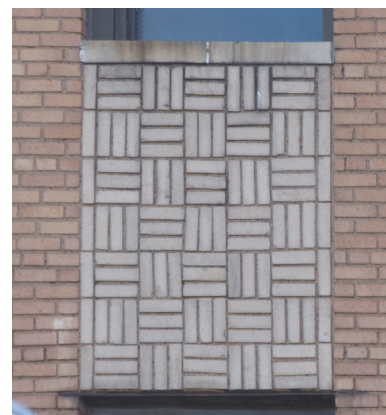
BRICK SPANDREL PATTERN
