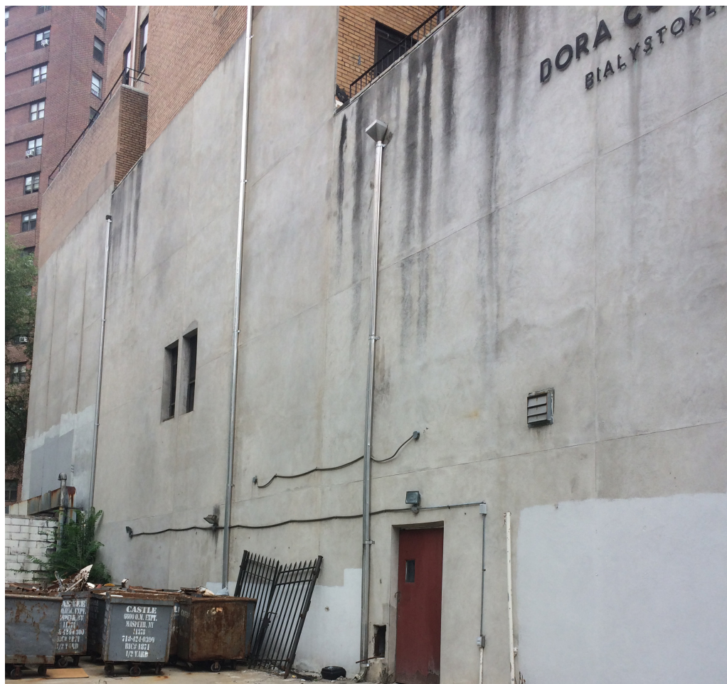
Exposed West Facade at Base
