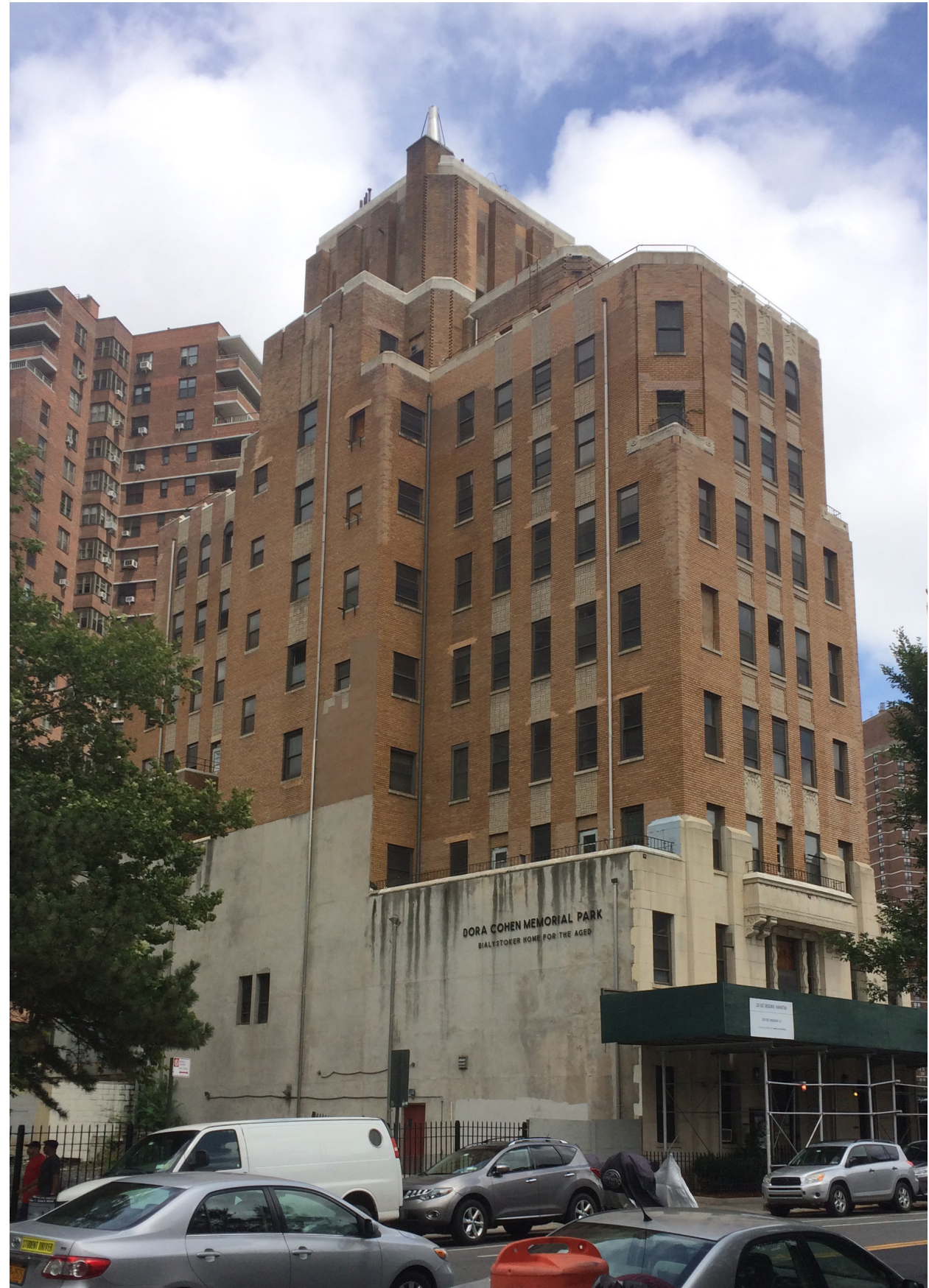
Existing West Facade
