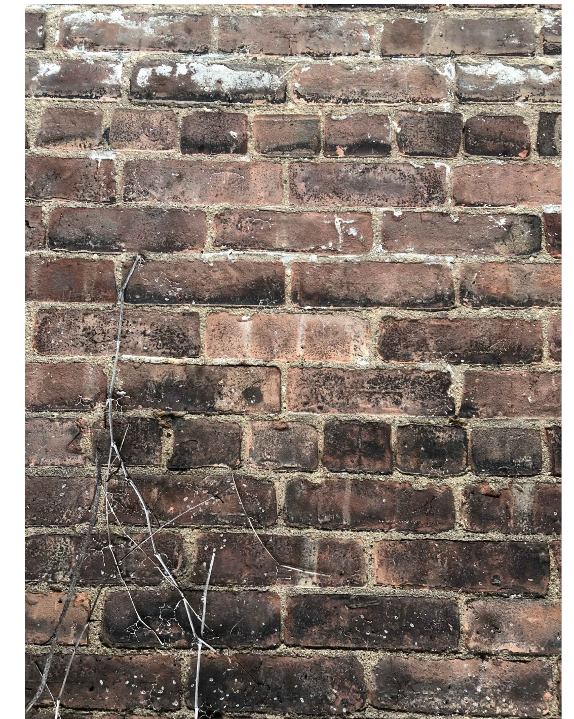
EXISTING REAR BRICK FACADE
