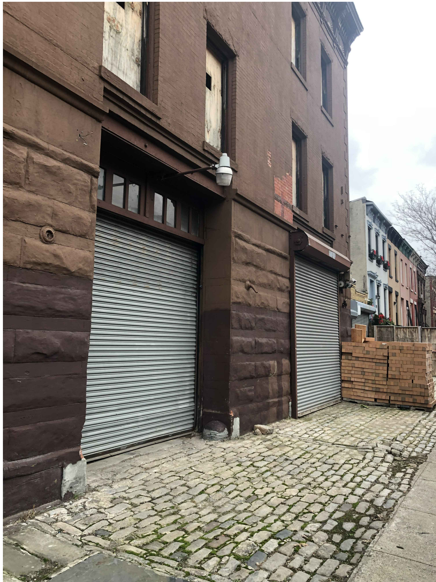
EXISTING MASONRY OPENING AND FIXED WOOD AND GLASS TRANSOM
