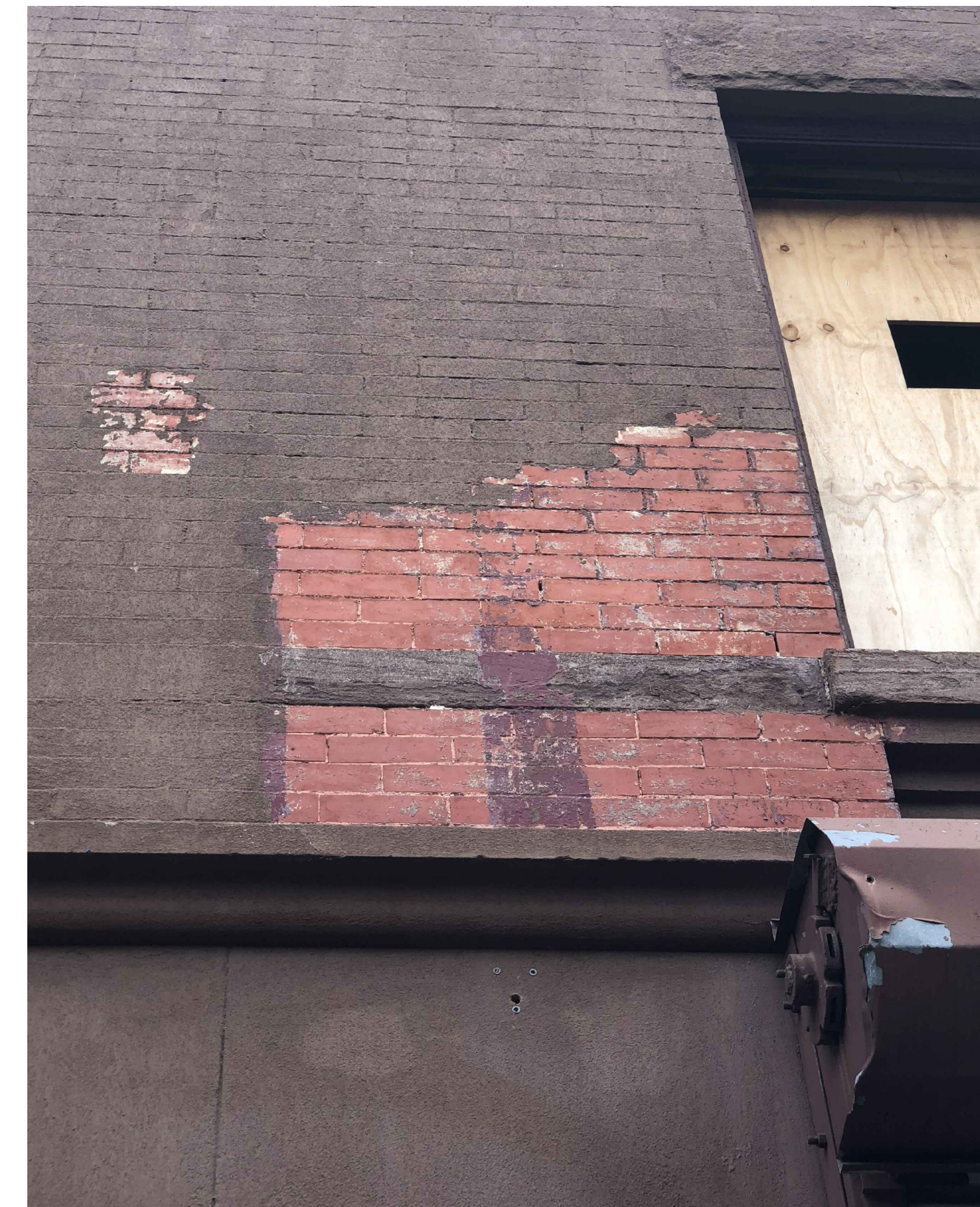
PAINT REMOVAL PHOTO AT EXISTING BUILDING
