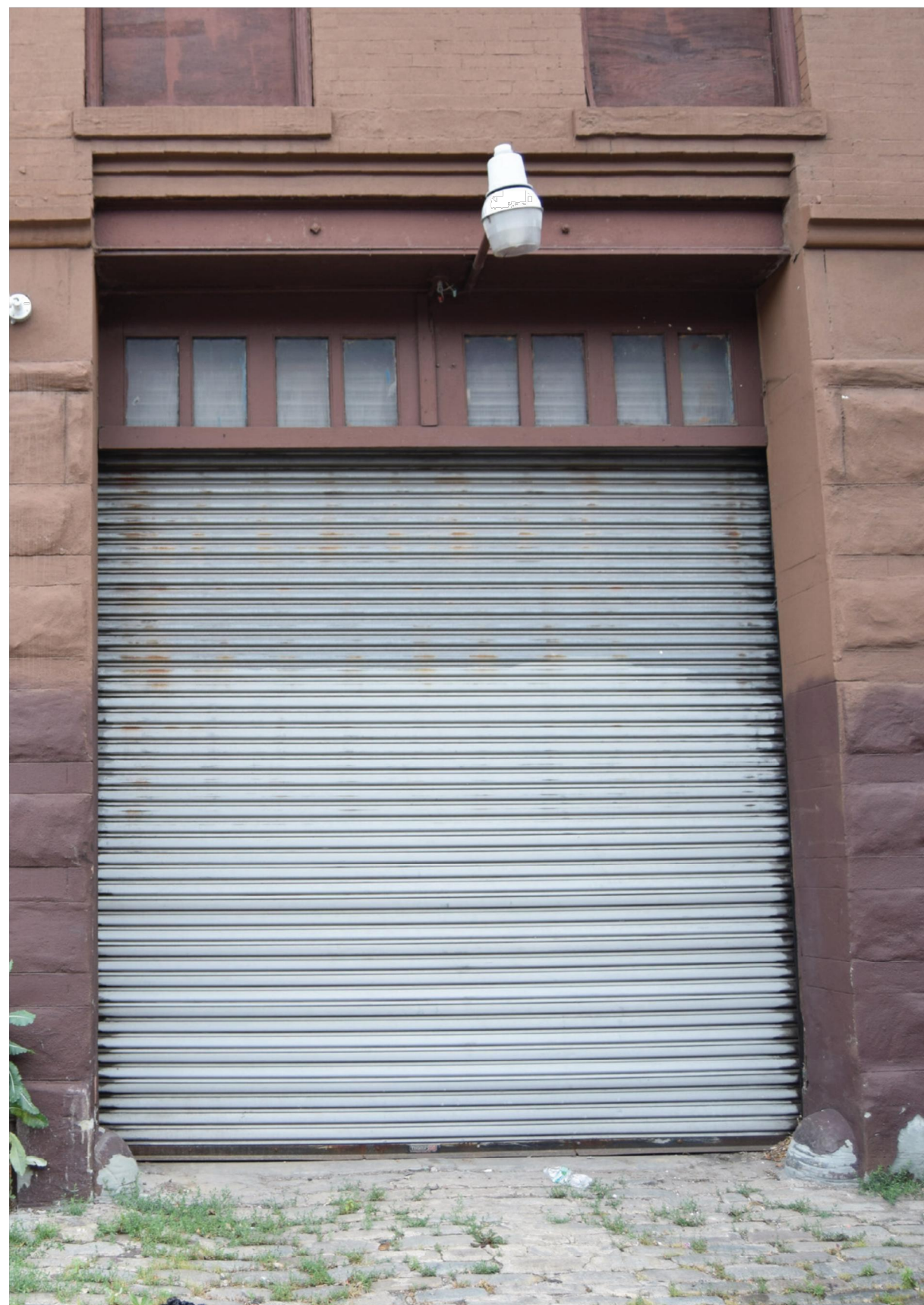
EXISTING MASONRY OPENING AND FIXED WOOD AND GLASS TRANSOM
