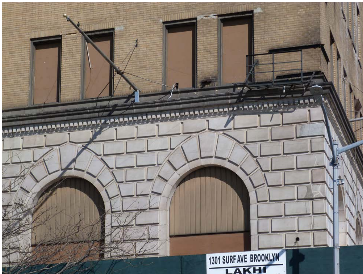
South Elevation, 2 nd & 3 rd Floors
