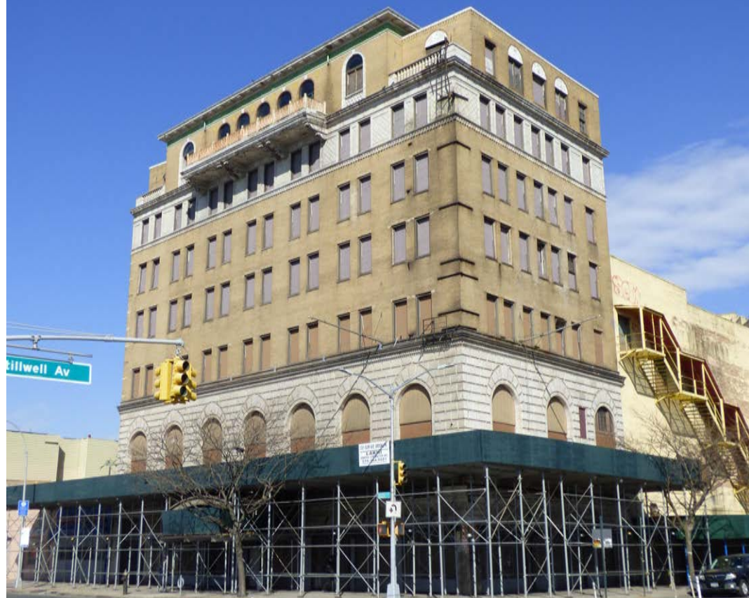
View to northwest from Surf & Stillwell Avenues
