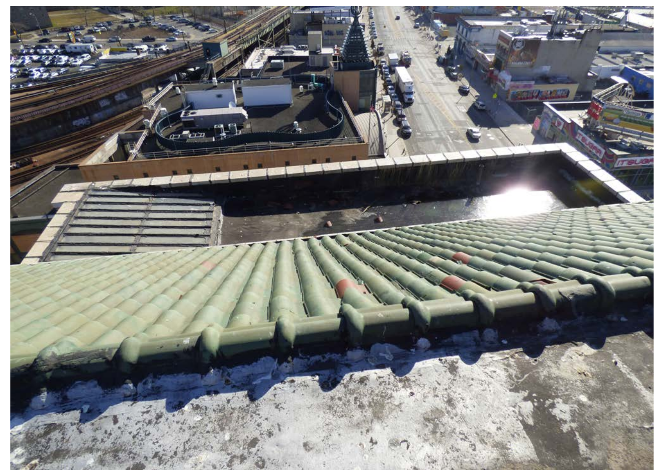
View to East over lower roof
