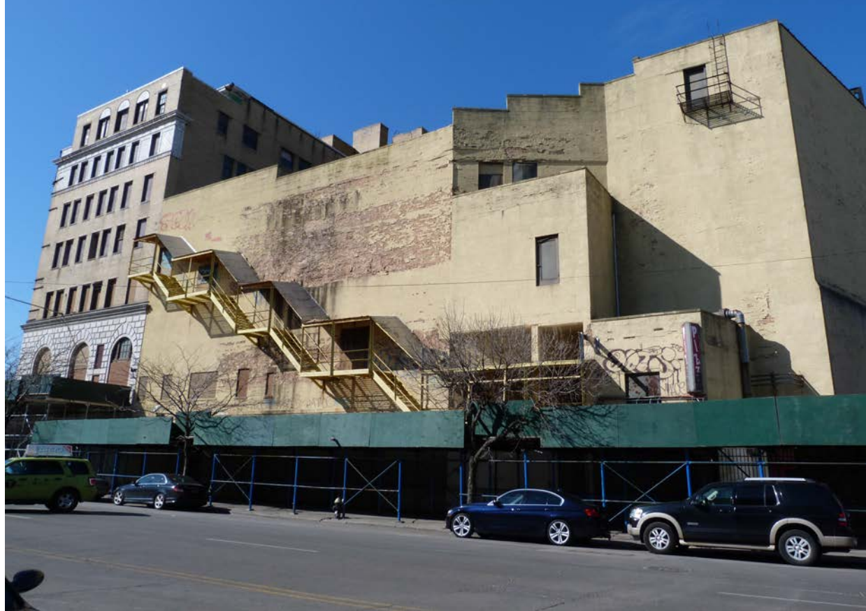
East Elevation overlooking Stillwell Ave.
