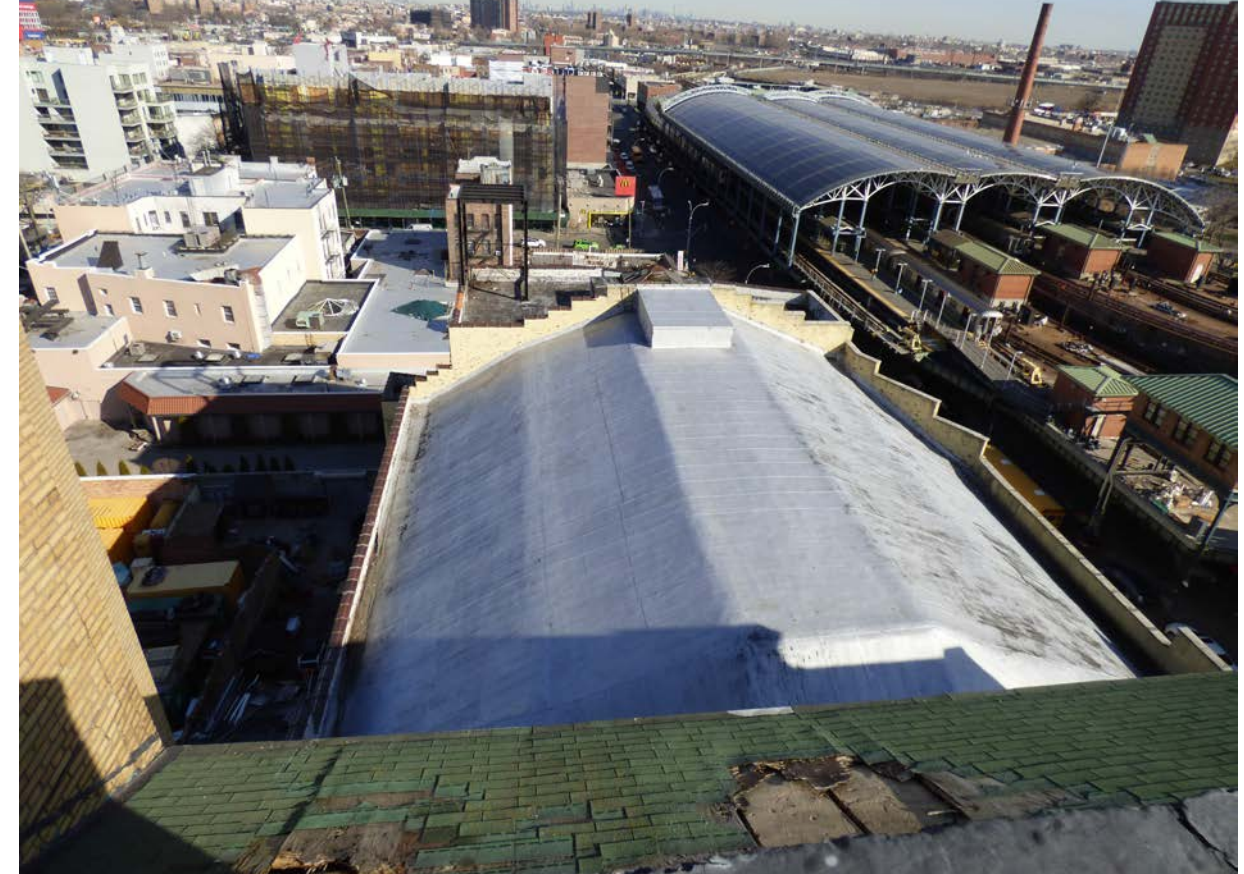
Roof View from rear of office building roof
