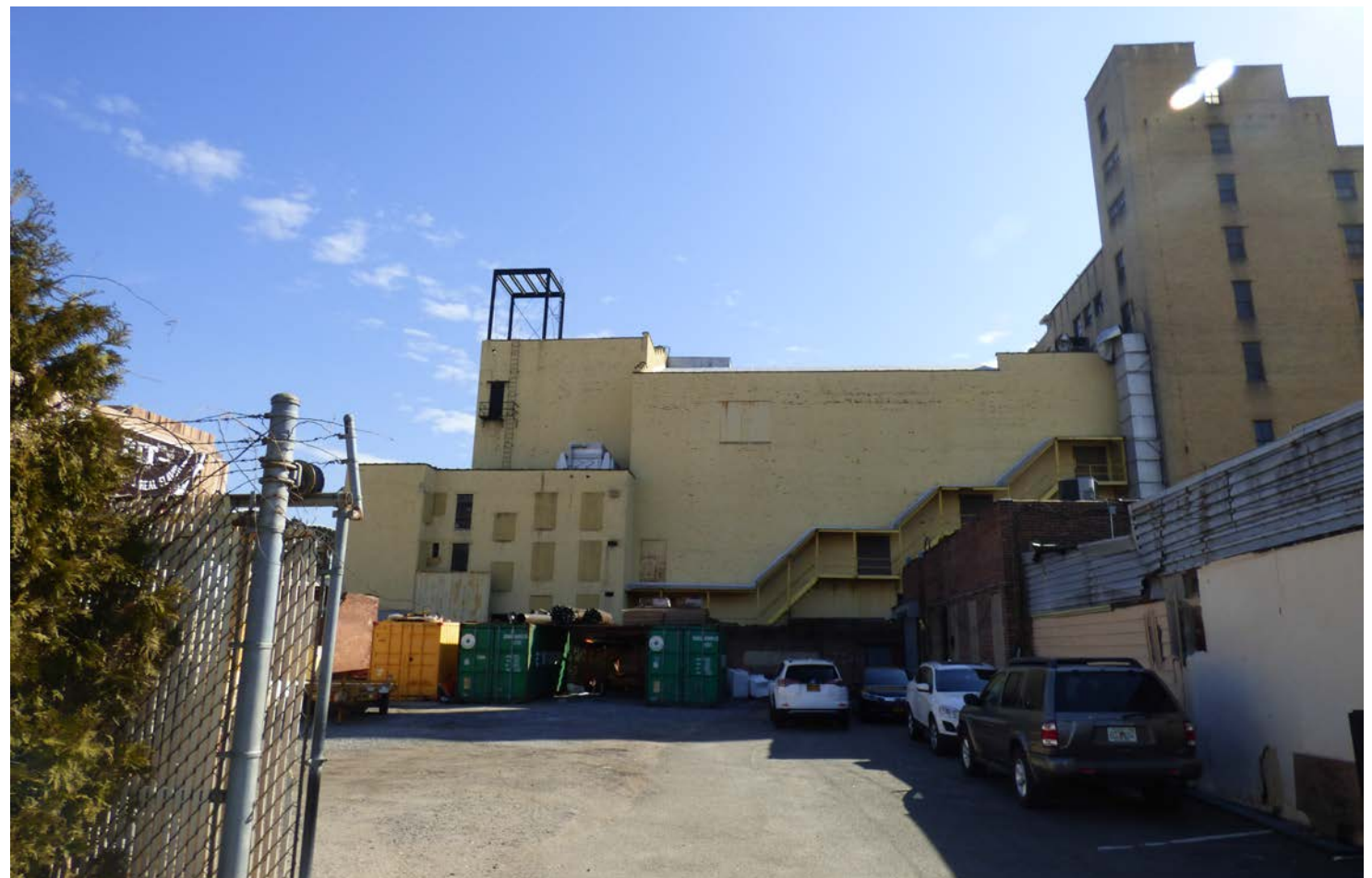
View east across neighboring lots to west elevation
