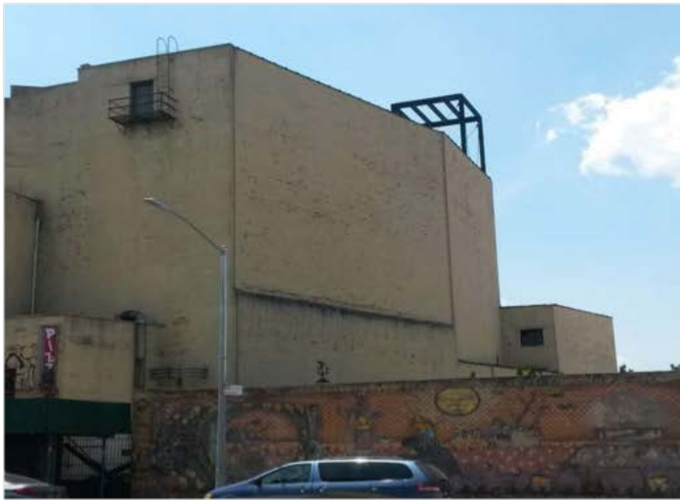
Figure 5 – North theater façade exterior wall
