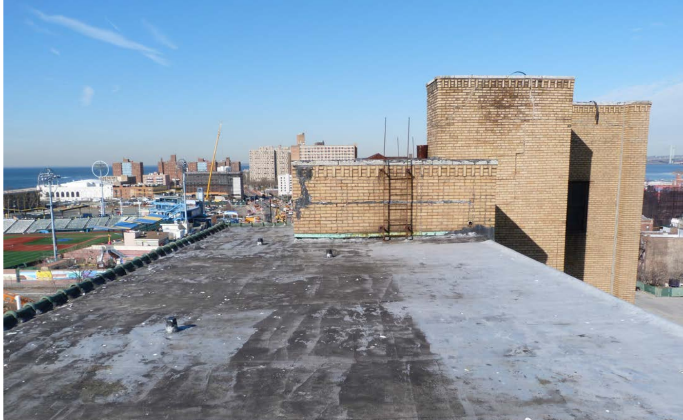
View to West over main roof
