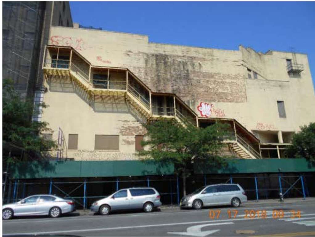
Figure 1 – East façade exterior stair.
