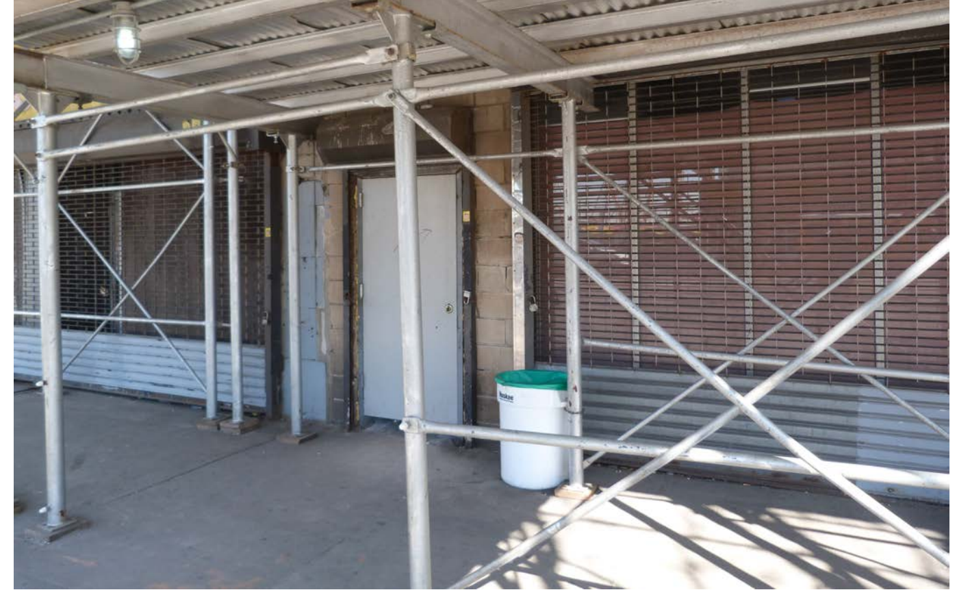
Altered infill under marquee
