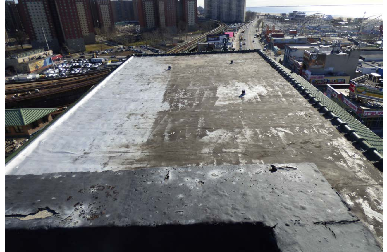
View to East over main roof
