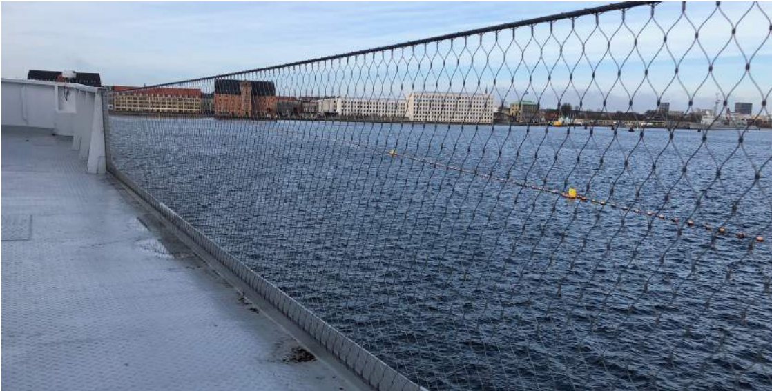
WIRE MESH + CABLE RAILING JAKOB ROPE SYSTEMS STAINLESS STEEL CABLING MESH WITH TOP / BOTTOM CABLE TAUT BET. STEEL POSTS BEHIND PARAPET
