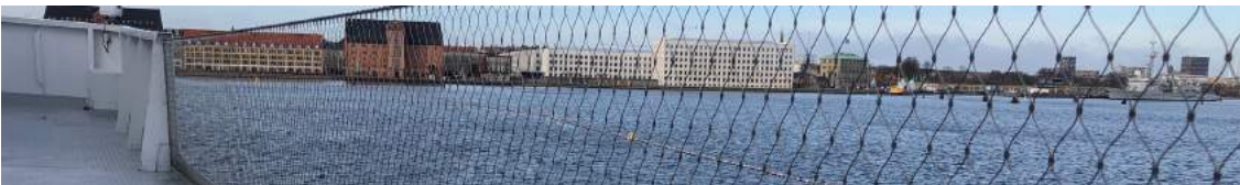
WIRE MESH + CABLE RAILING JAKOB ROPE SYSTEMS STAINLESS STEEL CABLING MESH WITH TOP / BOTTOM CABLE TAUT BET. STEEL POSTS BEHIND PARAPET
