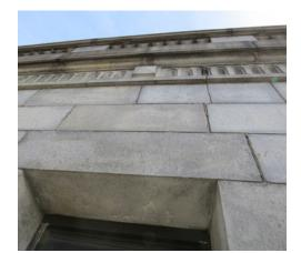
EXISTING CONDITIONS OF EXTERIOR GRANITE (SOILING AND CRACKING)
