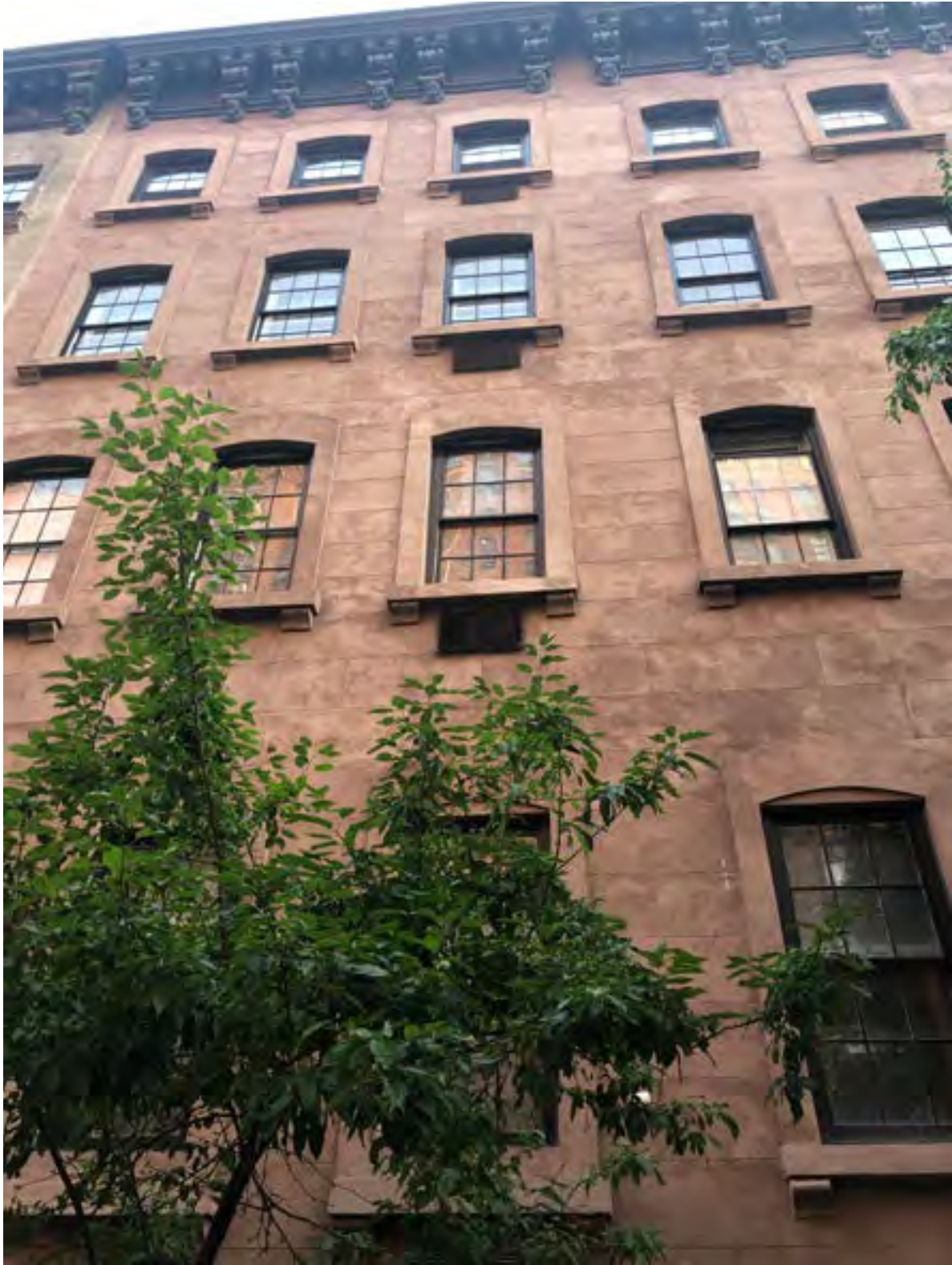
258 WEST 23RD STREET, EXAMPLE OF THRU-WALL GRILLES
