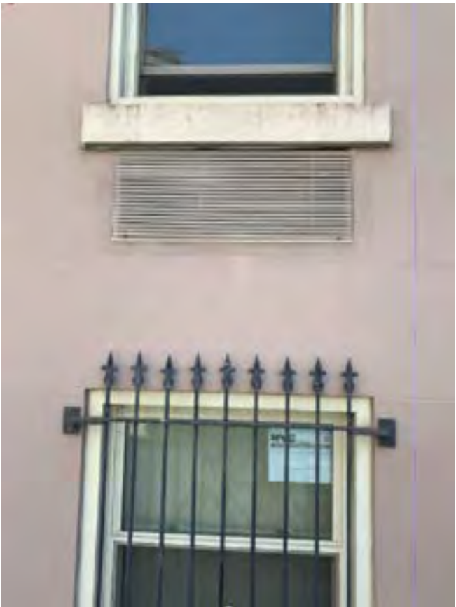
330 WEST 23RD STREET - EXAMPLE OF LOUVER THAT IS PAINTED SAME COLOR AS FACADE. THIS ONE IS ALMOST FLUSH WITH THE FACADE AS WELL. WE PROPOSE TO INSALL A LOUVER THAT IS COMPLETELY FLUSH WITH THE FACADE.
