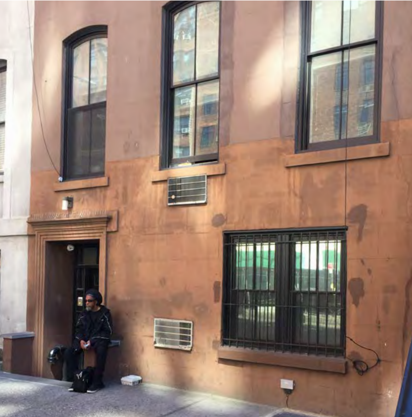
466 WEST 23RD STREET - THRU-WALL GRILLES
