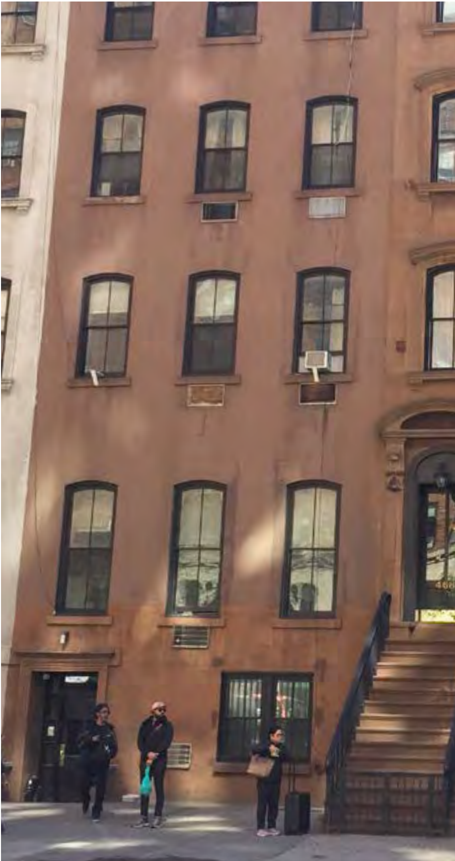
466 WEST 23RD STREET - THRU-WALL GRILLES
