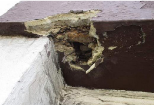
PROBES THROUGH REINFORCED STUCCO SYSTEM REVEALING ORIGINAL BROWNSTONE LINTELS AND SILLS
