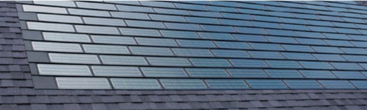
EXAMPLE OF “SUNTEGRA” SOLAR SHINGLE INSTALLED ON PITCHED ROOF PV PANELS REQUIRED BY CODE FOR BOTH HISTORIC BUILDING ROOFS.
