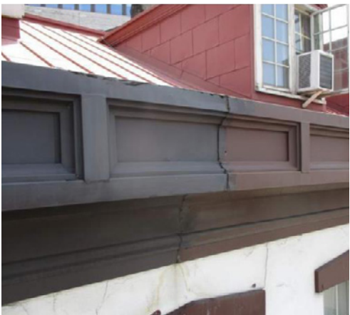
FORMED COPPER CORNICE OVER WOOD AND “NEW” BRICK STRUCTURE.
