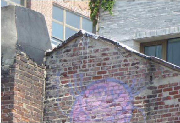
WEST FAÇADE. DELAMINATING AND SPALLED BLUESTONE COPING STONES.
