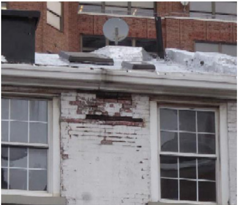
EXPOSED DETERIORATED NAILER WOOD OF THE FASCIA BOARD IMPACTING THE STABILITY OF THE ADJACENT MASONRY.
