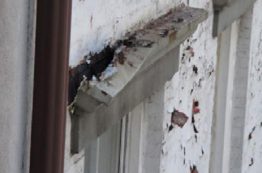
SHEET METAL COVER OVER BROWNSTONE LINTEL
