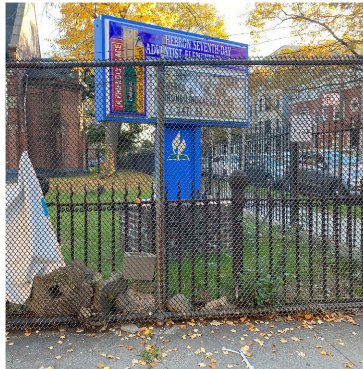
5. Chain link fence on top of historic fence.
