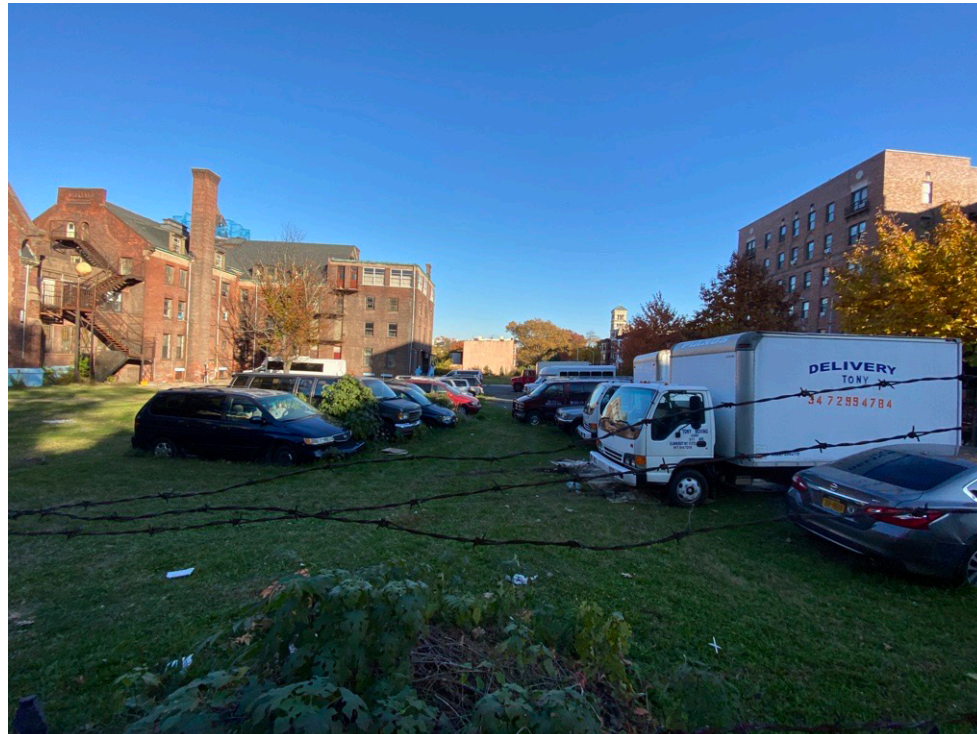
4. Barbed Wire on top of historic fence, cars parked on grass.
