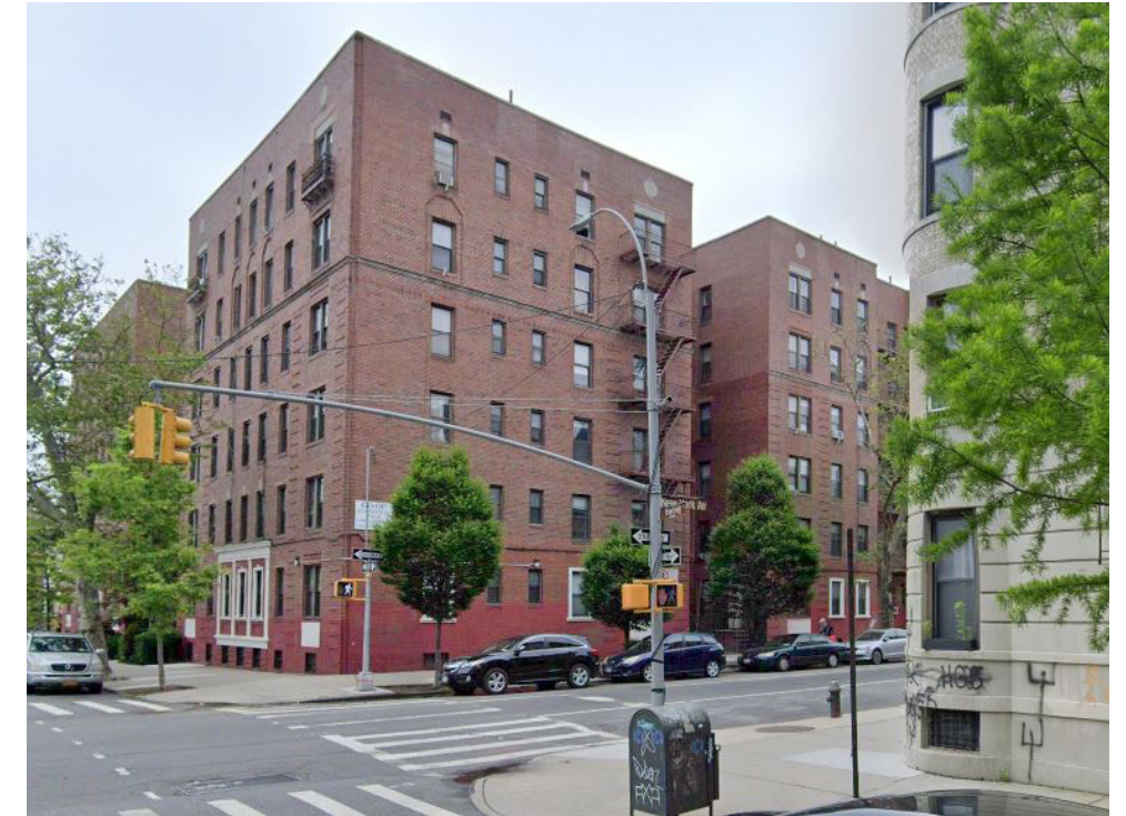
3. 960 Sterling Place (69 ft high, 170 ft long, 120 ft wide)
