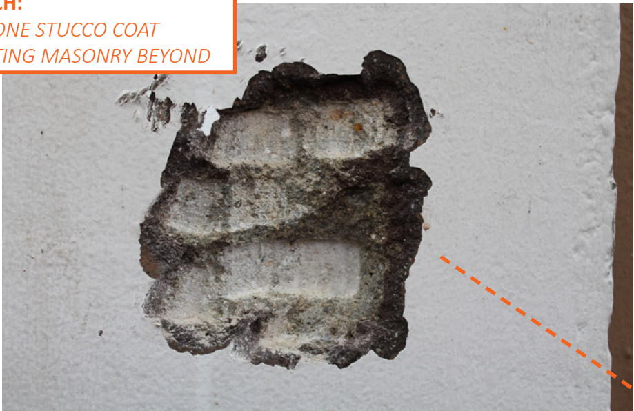
PAINT + BROWNSTONE STUCCO COAT - 1.25" CONCRETE SUBSTRATE - 1.5" EXISTING BRICK MASONRY BEYOND
