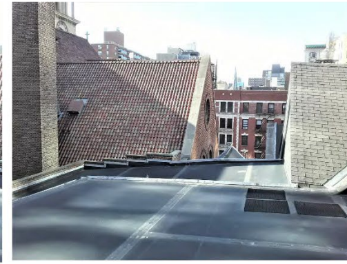
4. ROOF ABOVE APARTMENT 2 WITH ROOF ABOVE CLASSROOM 301 BEYOND LOOKING SOUTH
