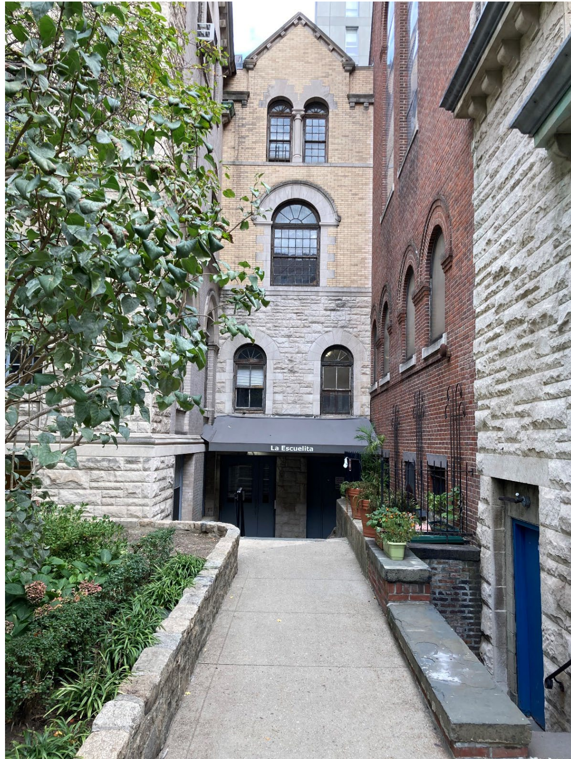
Existing Lower Level Entry
