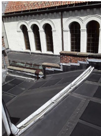
5. ROOF ABOVE STAIR 2 AND CLASSROOM LOOKING NORTHEAST
