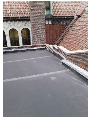
7. ROOF ABOVE CLASSROOM 301 AND CLASSROOM LOOKING EAST
