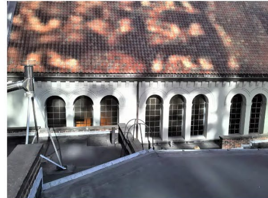
2. ROOF ABOVE APARTMENT 1 AND APARTMENT 2 LOOKING EAST
