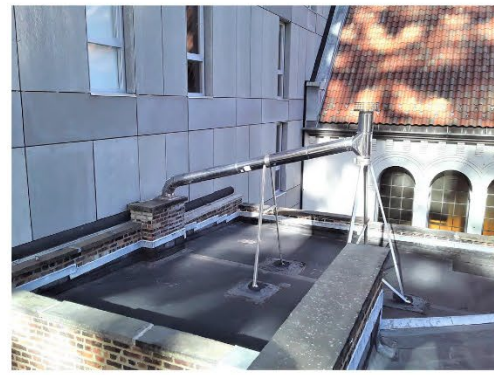
1. ROOF ABOVE APARTMENT 1 LOOKING EAST
