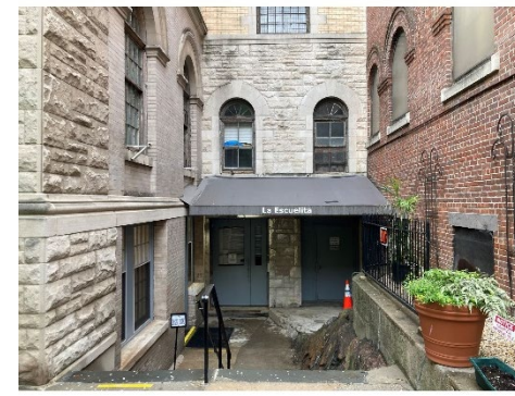
ENTRY CREASE VIEW LOOKING NORTH
