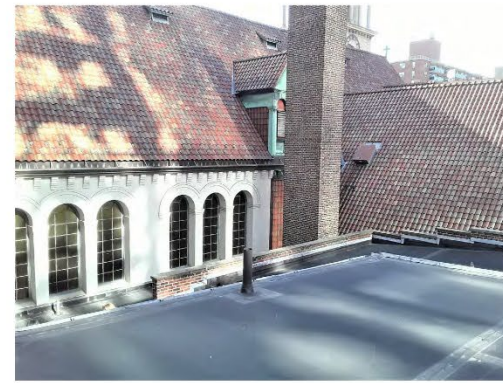
3. ROOF ABOVE CLASSROOM 301 LOOKING SOUTHEAST
