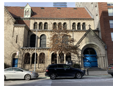
SANCTUARY BUILDING LOGGIA VIEW FROM AMSTERDAM
