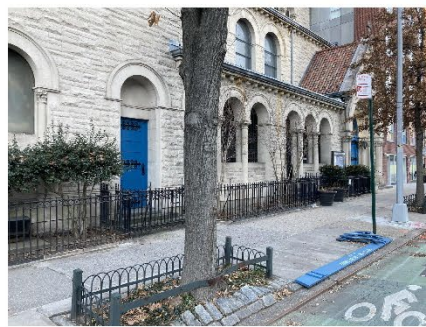
SANCTUARY BUILDING LOGGIA VIEW TO NORTHWEST
