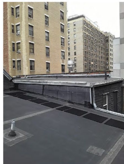
10. ROOF ABOVE CLASSROOM LOOKING NORTHWEST
