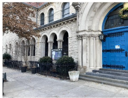
SANCTUARY BUILDING LOGGIA VIEW TO SOUTHWEST
