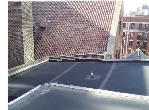
9. ROOF ABOVE CLASSROOM 301 LOOKING SOUTH
