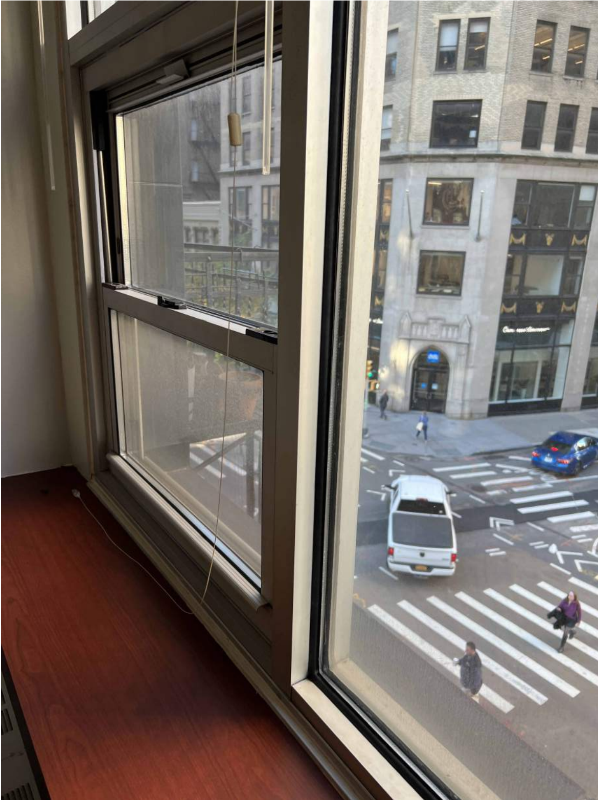
11 ALUMINUM FRAME INSULATED GLAZING WINDOWS DOUBLE HUNG WINDOW
