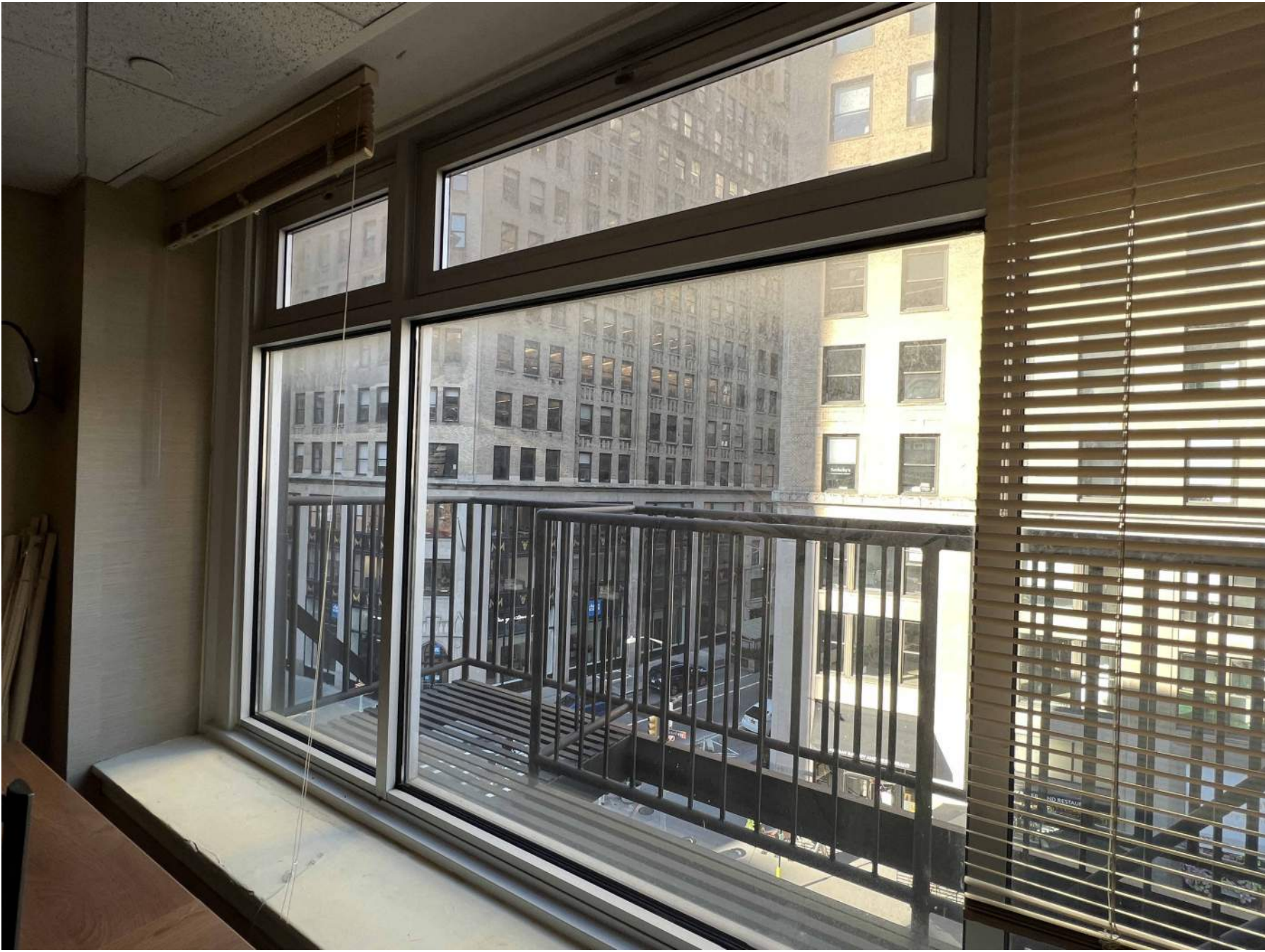
20 ALUMINUM FRAME INSULATED GLAZING WINDOWS 4TH FOOR WINDOWS MATCH THE LAYOUT ON APPROVED DRAWINGS.
