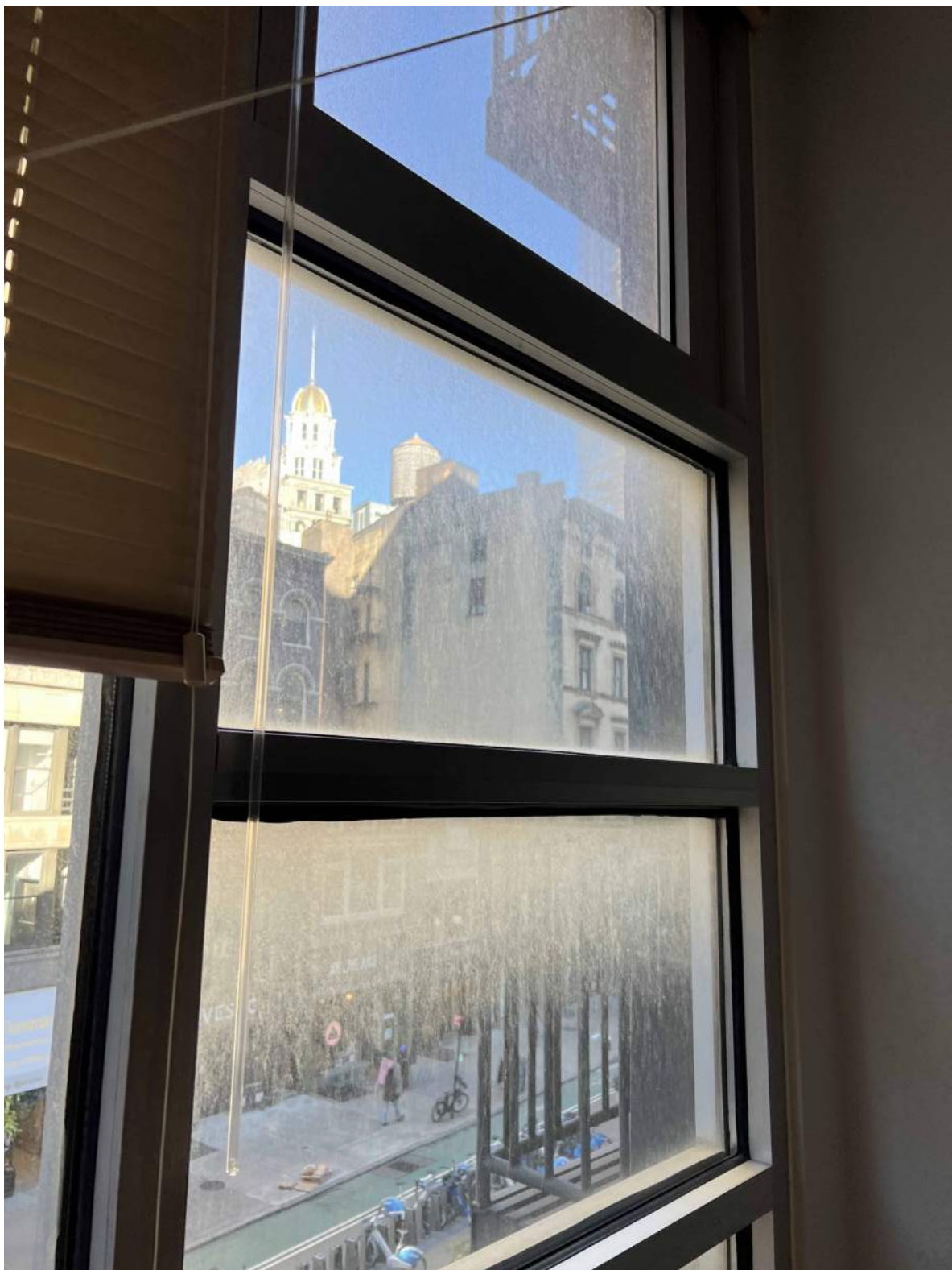
11 ALUMINUM FRAME INSULATED GLAZING WINDOWS WINDOWS ARE IN GOOD CONDITION
