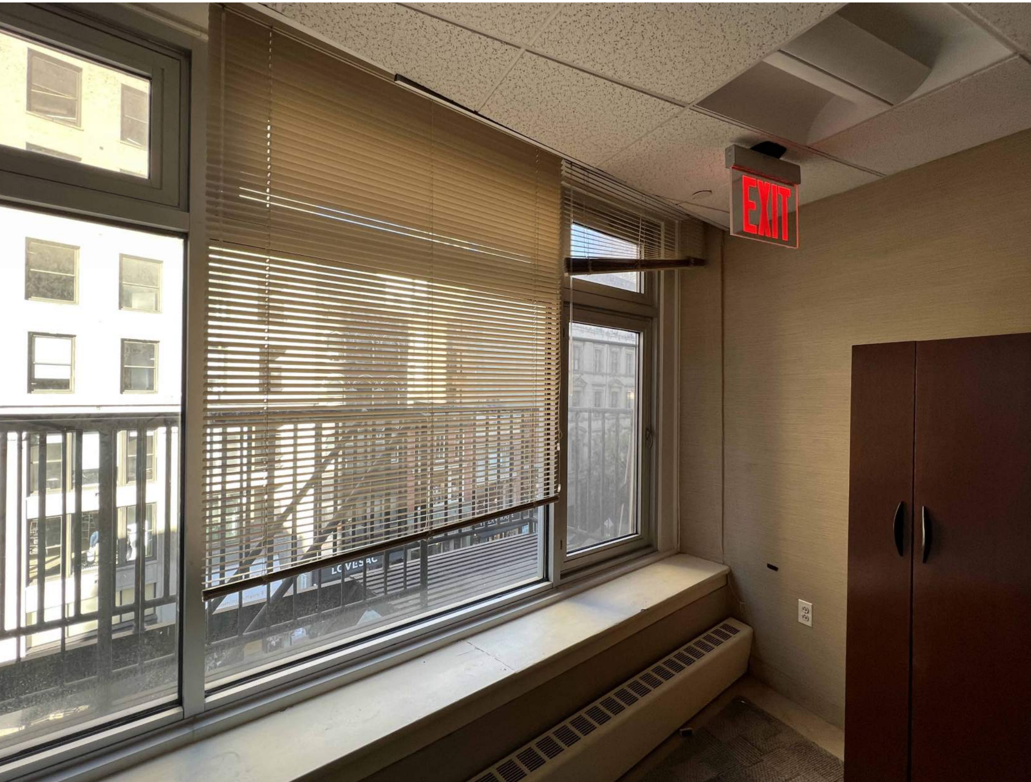
12 ALUMINUM FRAME INSULATED GLAZING WINDOWS WINDOWS ARE IN GOOD CONDITION
