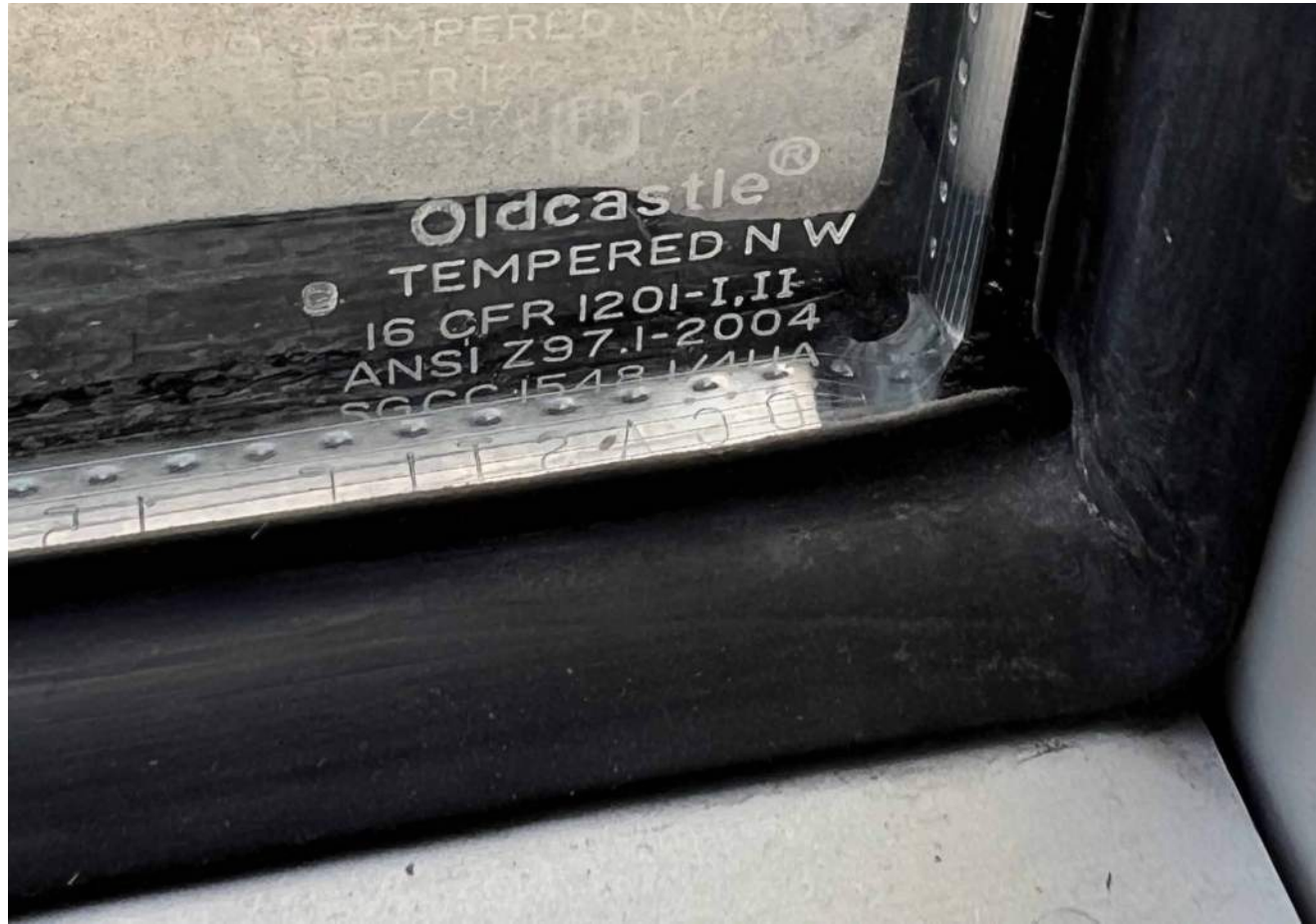
22 ALUMINUM FRAME INSULATED GLAZING WINDOWS WINDOWS ARE IN GOOD CONDITION
