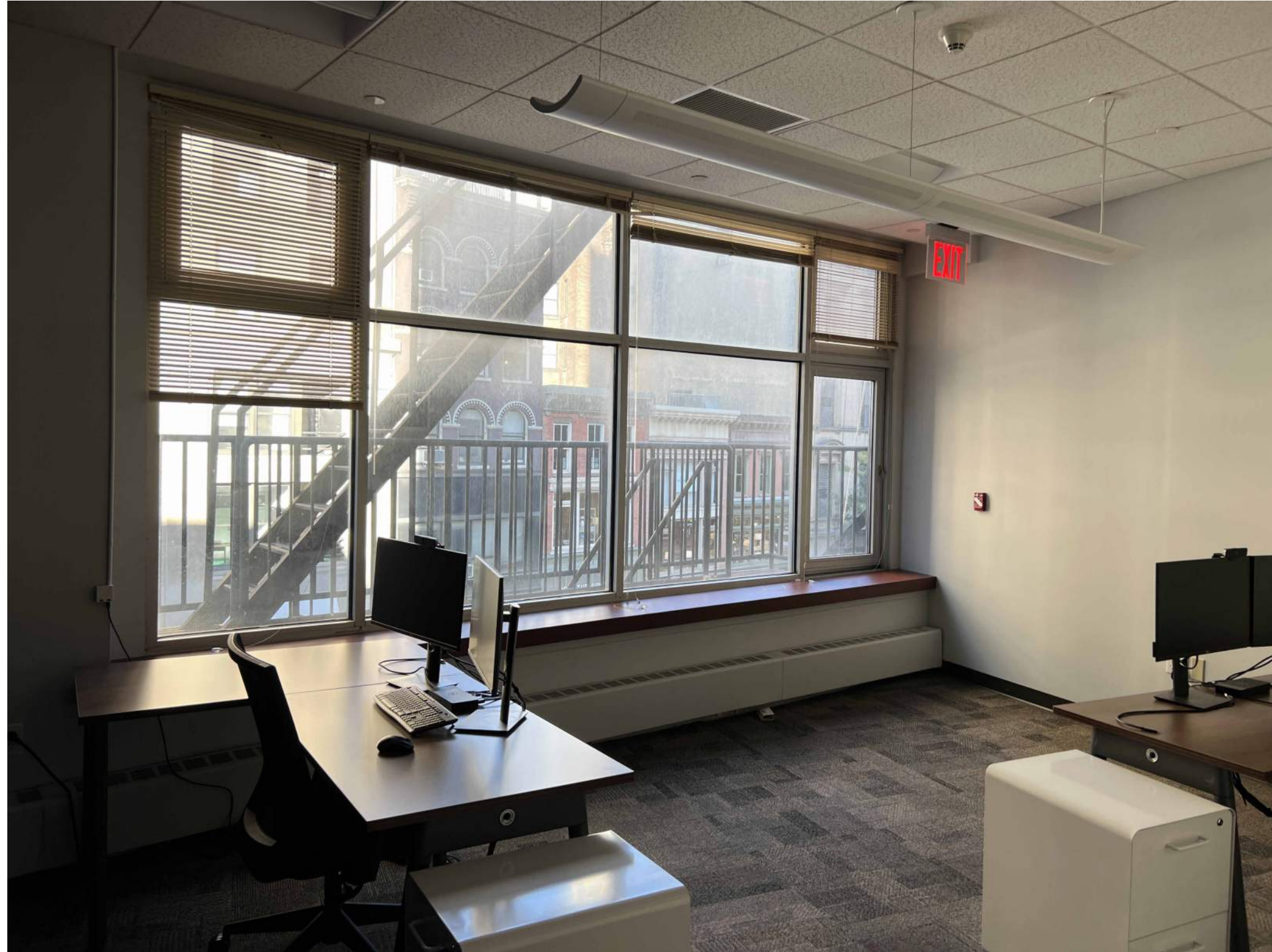
12 ALUMINUM FRAME INSULATED GLAZING WINDOWS WINDOWS ARE IN GOOD CONDITION - 3RD FLOOR WINDOWS, NORTH BAY
