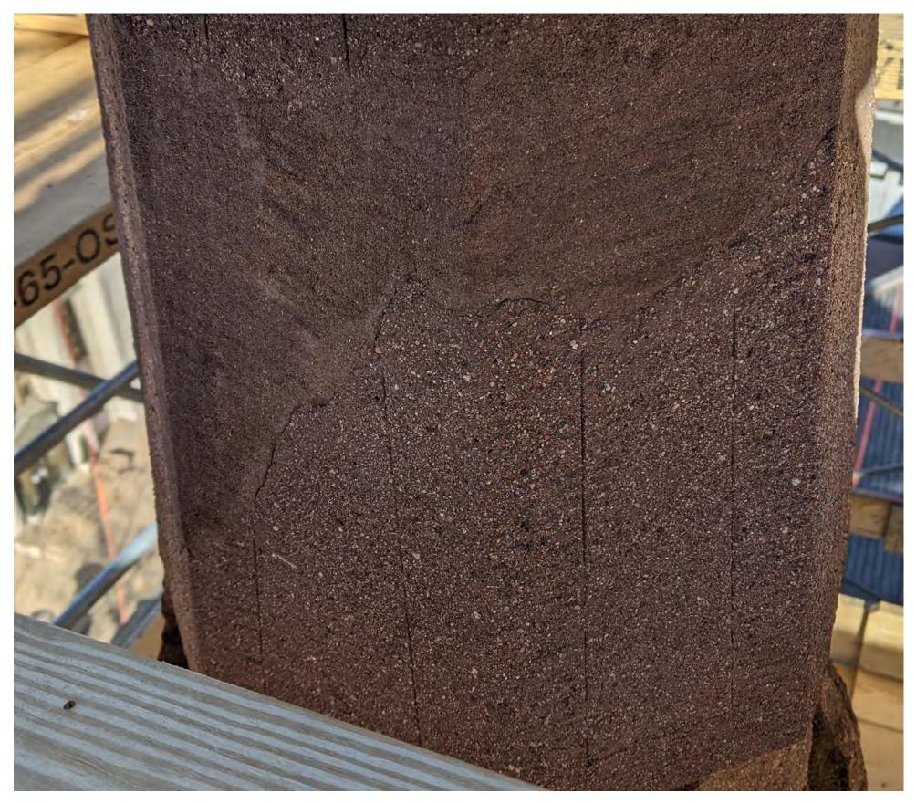
Stone Finials – Horizontal Cracks and Poor Repairs. EXISTING CONDITIONS
