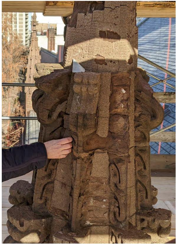
Stone Finials – Cracks, Spalls, Poor Repairs. EXISTING CONDITIONS
