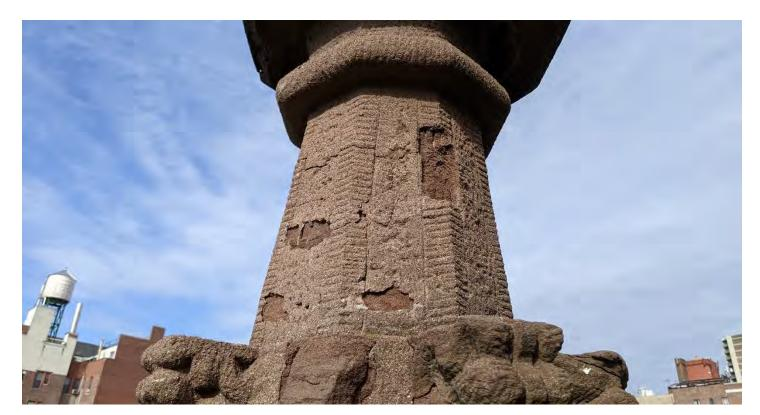
Stone Finials – Resurfacing Failures.
