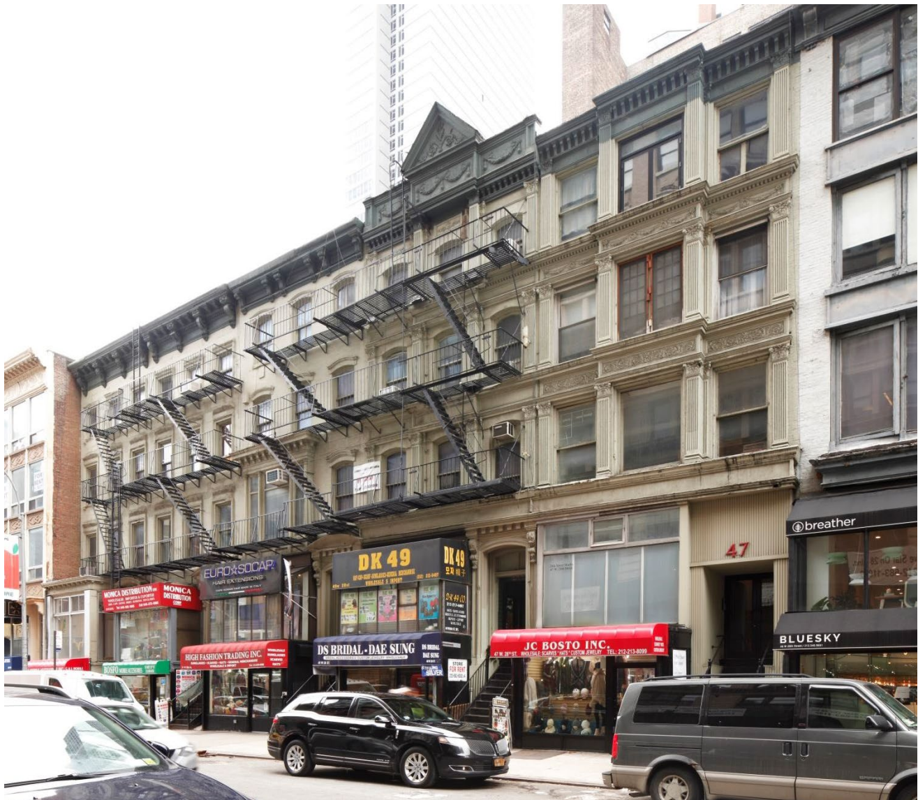
47-55 West 28th Street, Landmarks Preservation Commission, 2019
