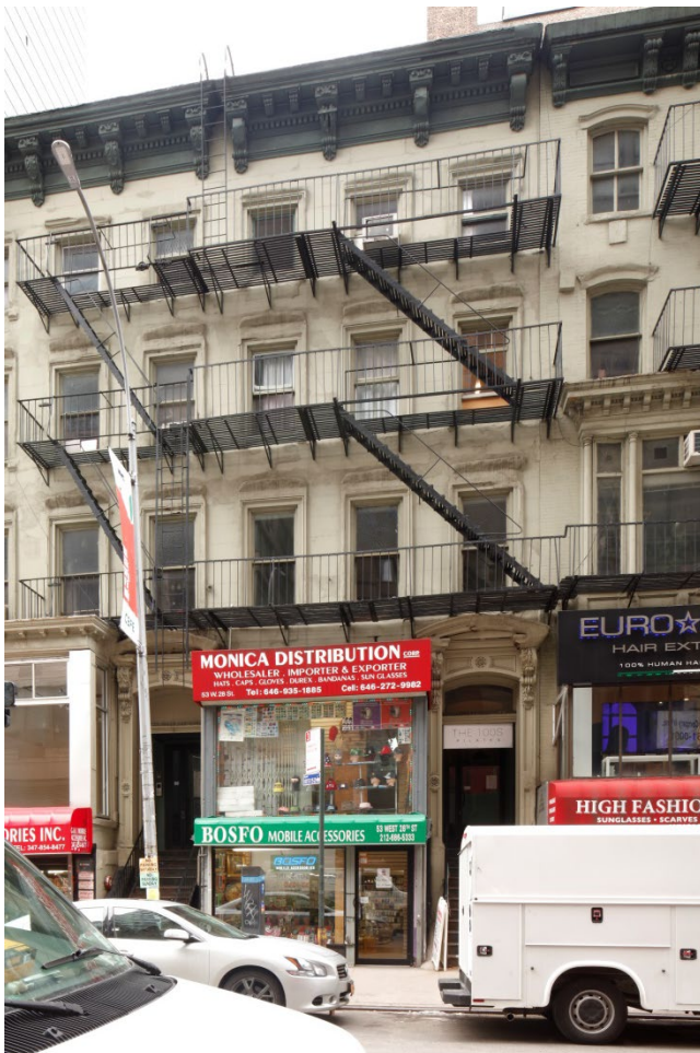
53 West 28th Street, Landmarks Preservation Commission, 2019
