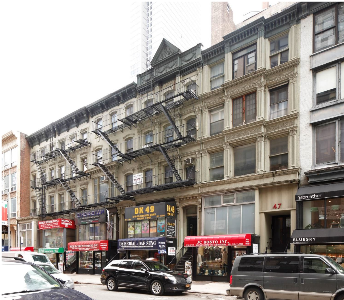
47-55 West 28th Street, Landmarks Preservation Commission, 2019
