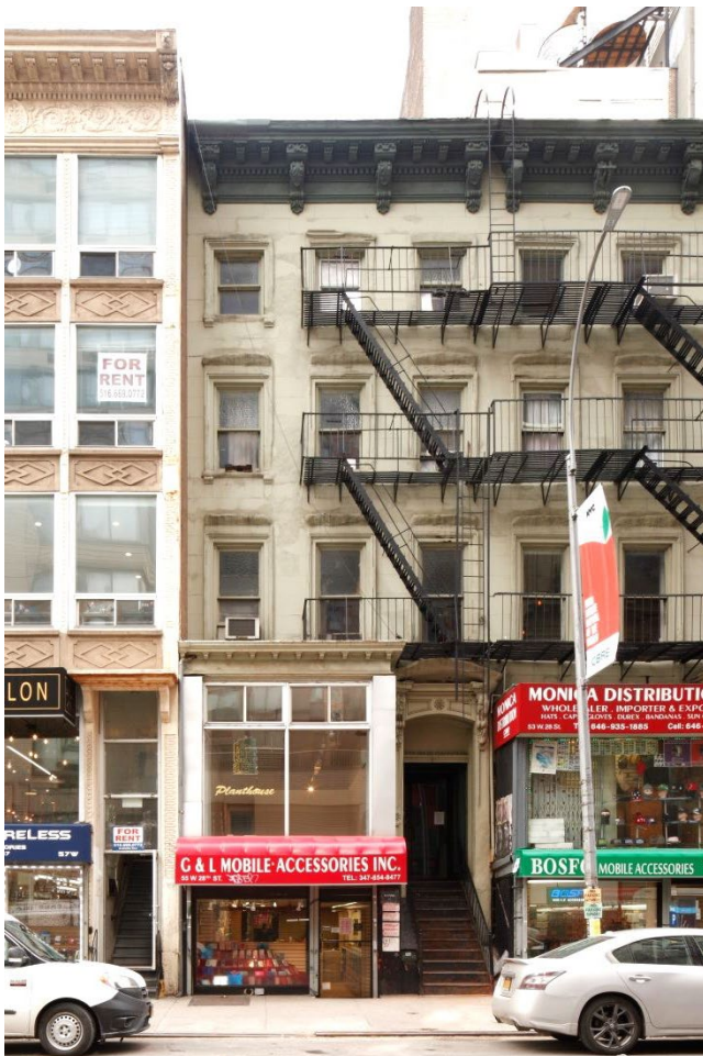
55 West 28th Street, Landmarks Preservation Commission, 2019
