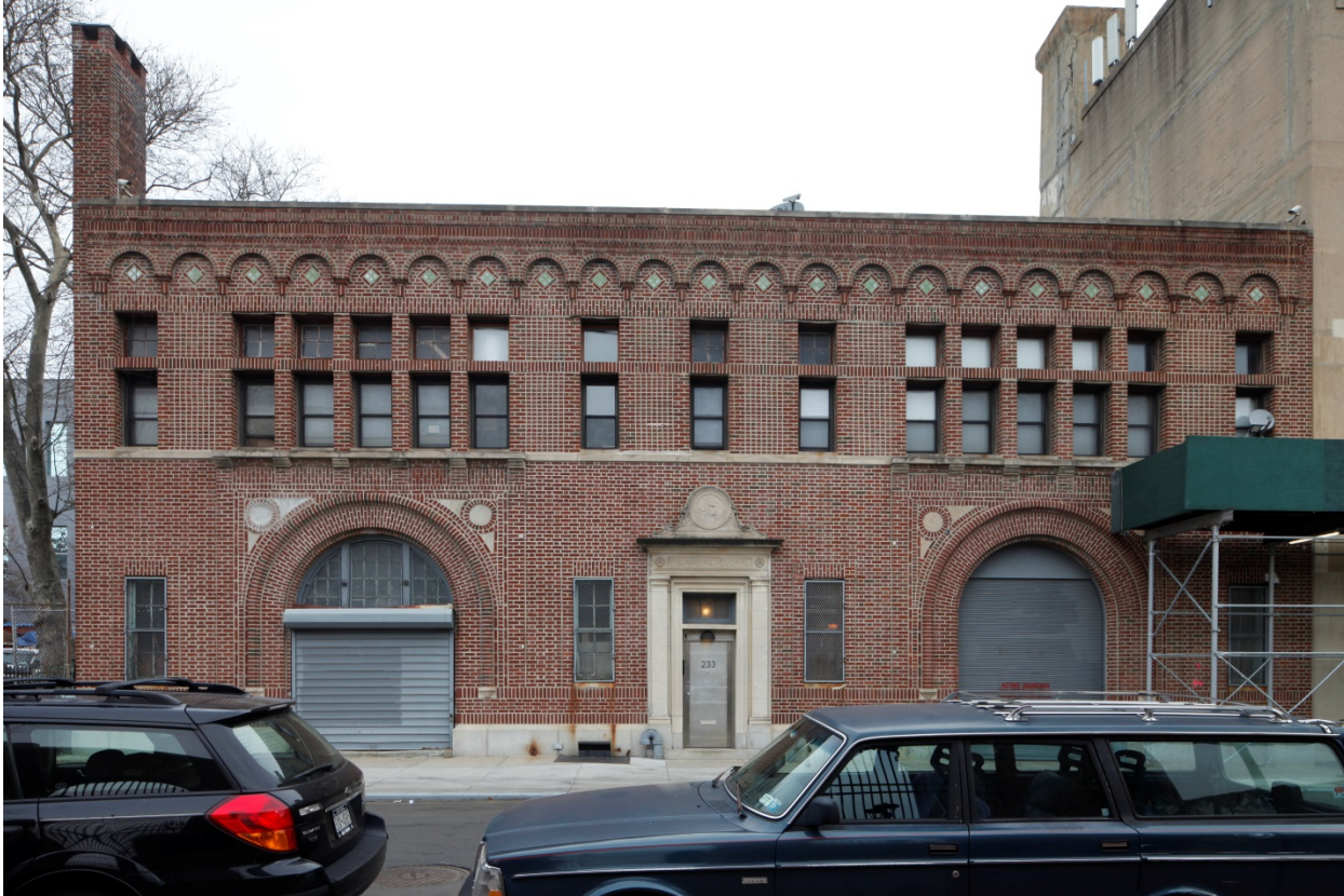
ASPCA Rogers Memorial Building, LPC, 2017
