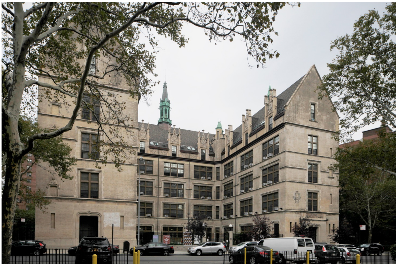
El Barrio's Artspace, previously PS 109, Barrett Reiter (LPC), October 2017
