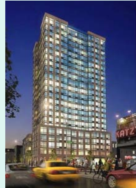
Ludlow St, LES (Edison Properties)
