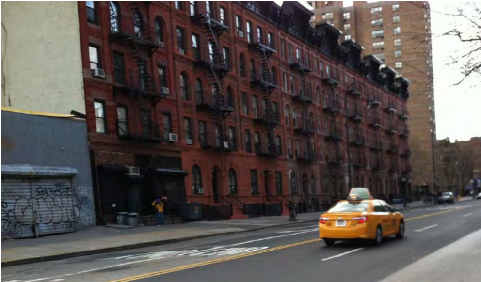
View Southwest toward Buildings #642 - 628
