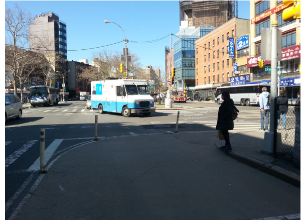
Painted curb extension, East Broadway at Pike St.
