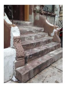
Figure 50: Poor Maintained Housing Entrance
