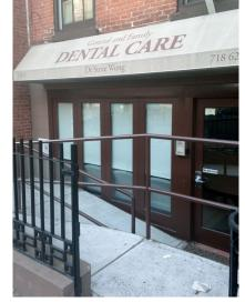
Figure 34: Example of Permanent Ramps
