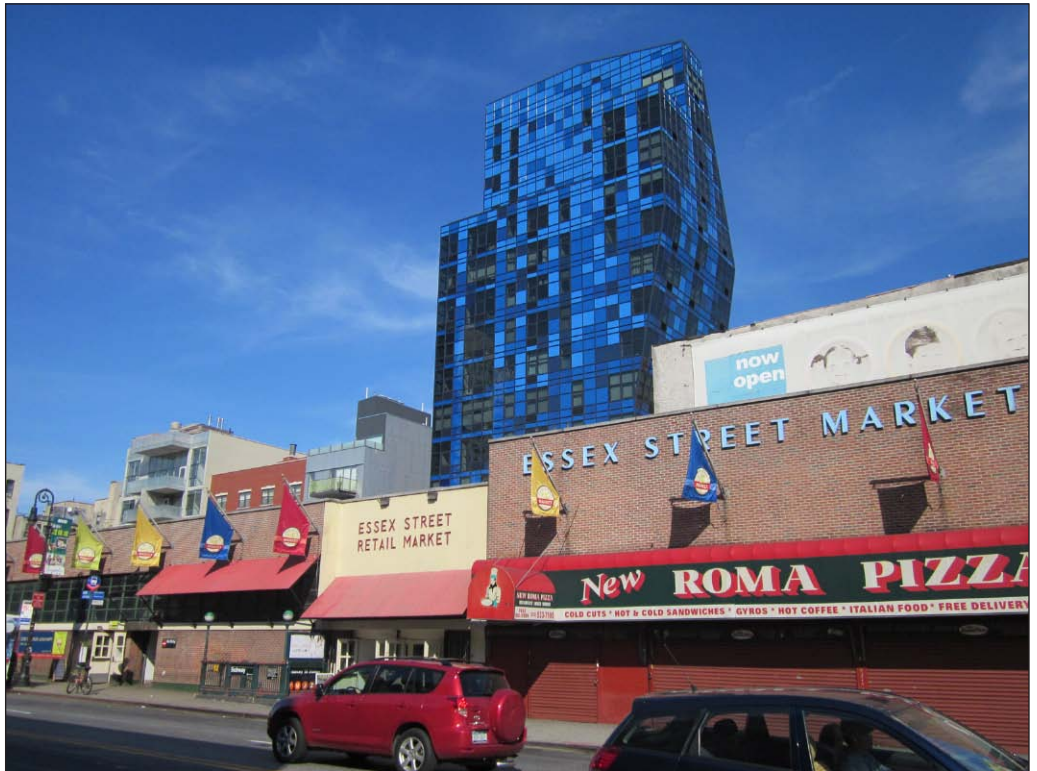
Site 9, looking east from just north of Delancey Street 13
