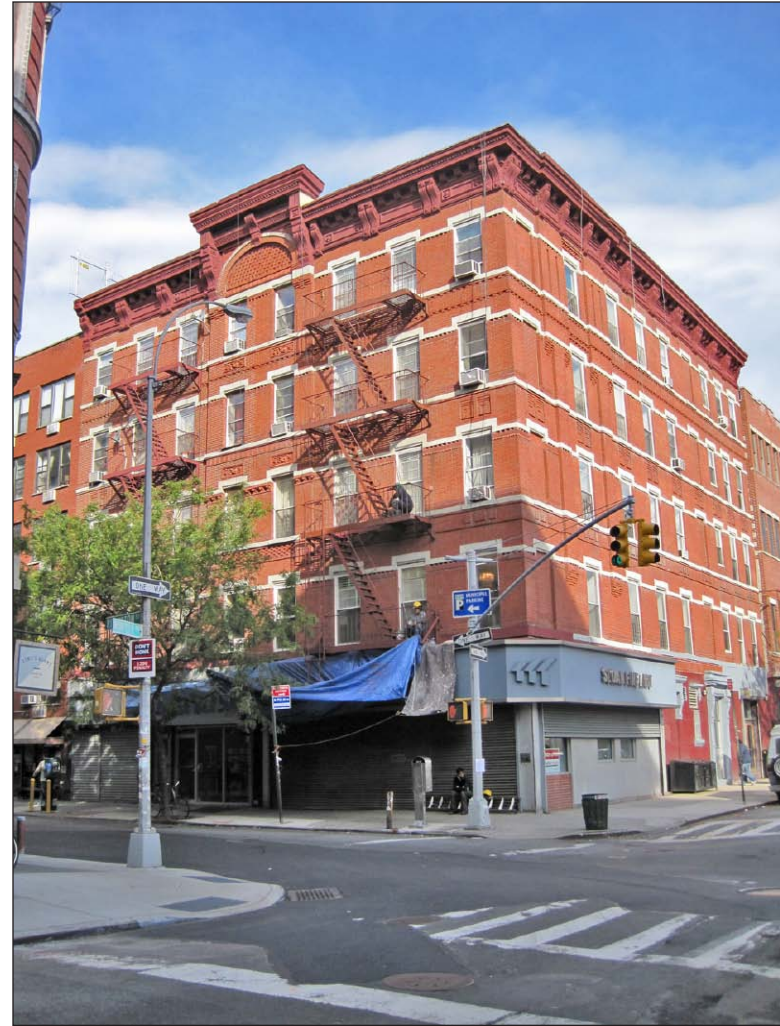
View northwest at Rivington and Norfolk Streets 17
