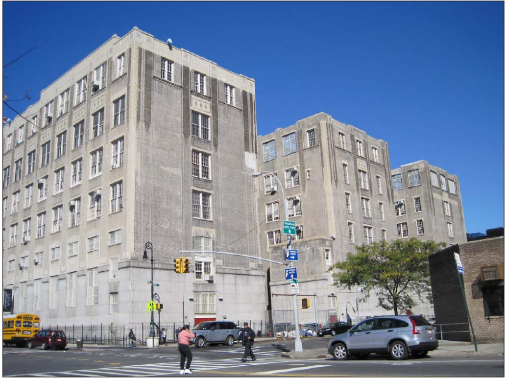
Seward Park High School, view northwest from Grand and Essex Streets 6
