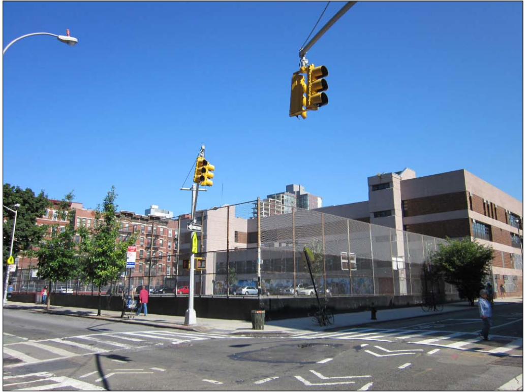
Lower East Side Preparatory School/Marta Valle School, 29 view northwest from Rivington and Suffolk Streets
