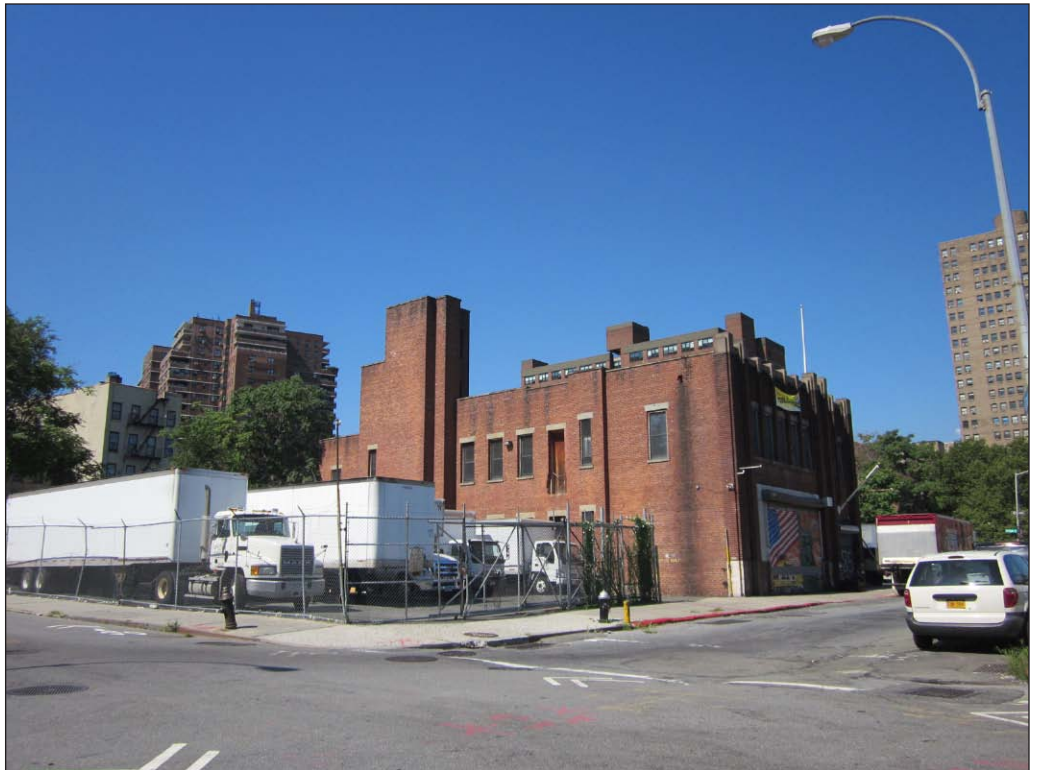
Site 5, looking southwest from Broome and Clinton Streets 8
