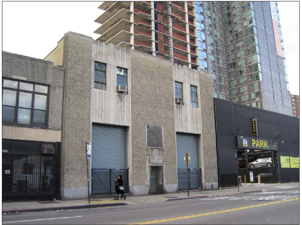
Substation 409 (#11), 163 Essex Street 26
