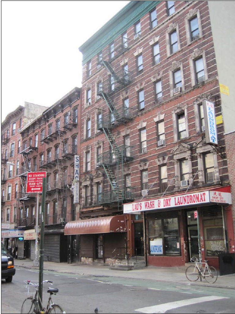
View southeast on Rivington Street from Essex Street 16
