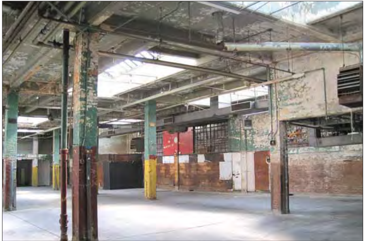
Interior - View southwest
